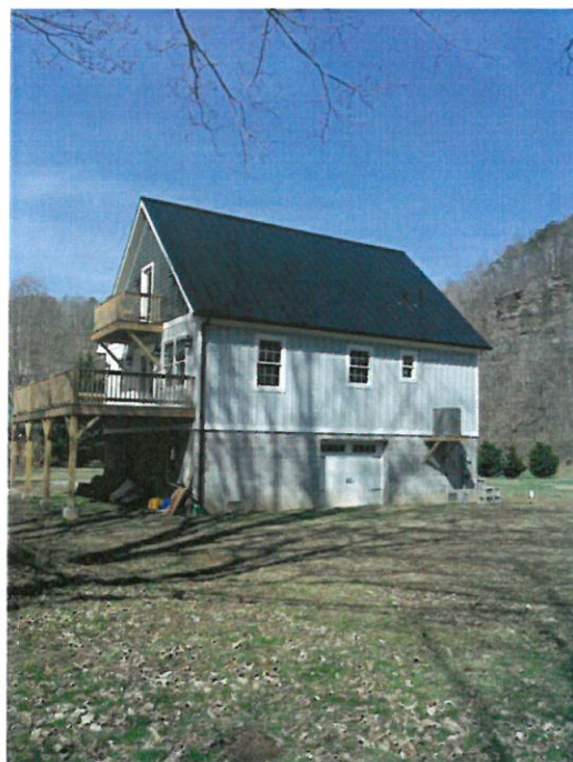
Rear of Structure -3/24/2016
