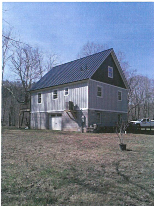
Rear and Left of Structure- 3/24/2016
