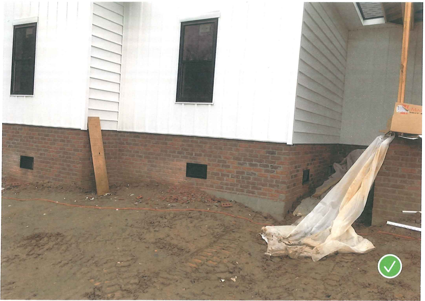
FLOOD VENTS IN GARAGE.JPG
