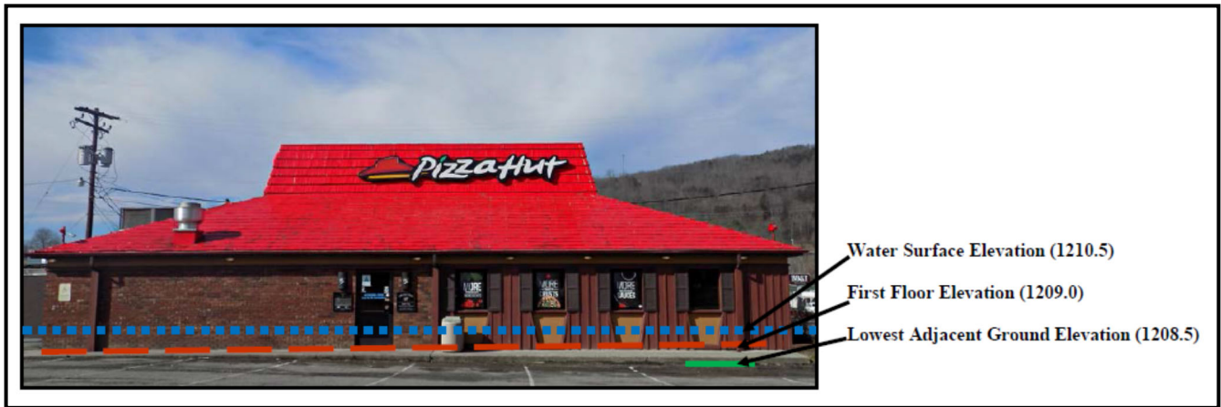
Figure A4: Example 2 Structure Data
