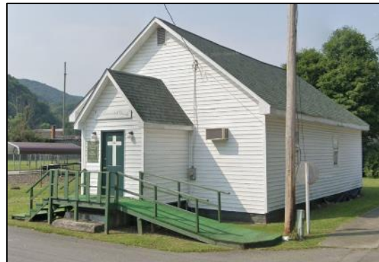
Figure 133. First Pentecostal Church, Highest non-historical community asset flood depth (3.3 ft) in Rainelle (Building ID: 13-13-0005-0081-0000_176 )
