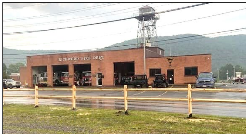
Figure 92. Richwood Volunteer Fire Department (Building ID: 34-06-0005-0407-0005_10 )
