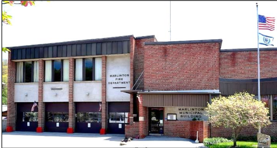
Figure 88. Marlinton Volunteer Fire Department (Building ID: 38-08-0001-0095-0000_709B )
