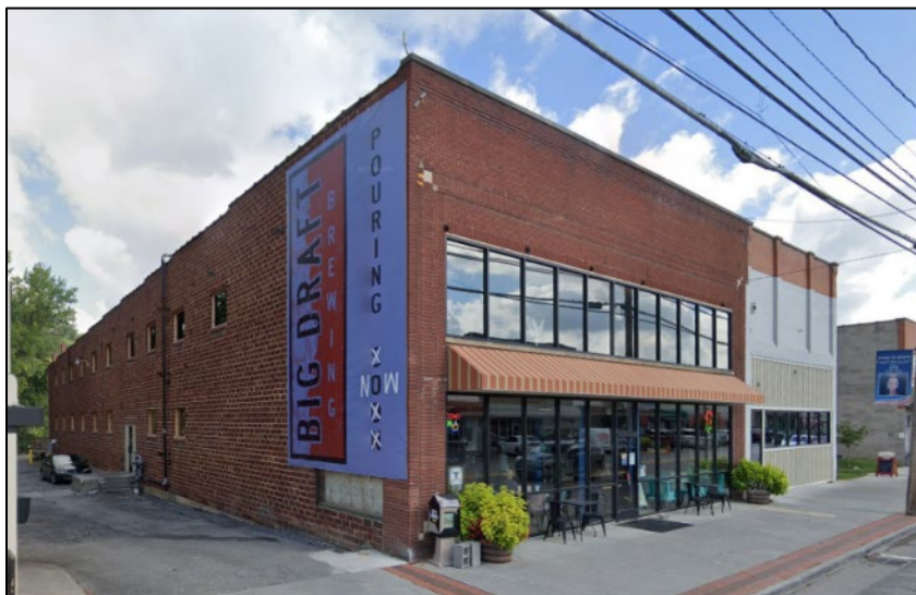
Figure 67. Structure with the maximum value ($1.68M) in floodplain of White Sulphur Springs (Building ID: 13-17-0008-0186-0000 703 )
