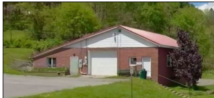
Figure 102. Camden-on-Gauley Police Department, Storage Facility (Building ID: 51-01-0003-0094-0000 9676 )
