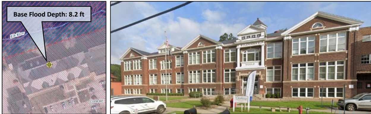
Figure 138. Highest estimated building loss in Clendenin ($84K), Clendenin Health Center (Building ID: 20-02-0007-0004-0003_107 )
