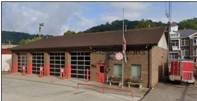
Figure 94. Clendenin Volunteer Fire Department (Building ID: 20-02-0007-0040-0000_109 )
