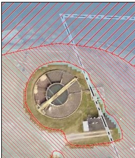
Figure 125. Richwood Wastewater Treatment Plant, Highest community asset value ($880K) in floodplain (Building ID: 34-05-0030-0014-0000_408 )
