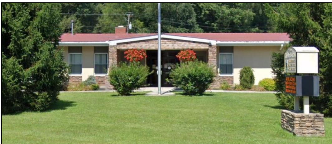
Figure 98. Rainelle Police Department (Building ID: 13-13-0004-0147-0000_1233 )
