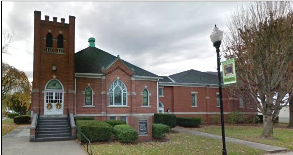
Figure 123. Marlington Presbyterian Church in floodway (Building ID: 38-08-0002-0104-0000_815 )
