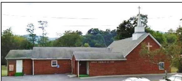
Figure 129. First Church of God in White Sulphur Springs' Floodway (Building ID: 13-17-0009-0066-0000 155 )
