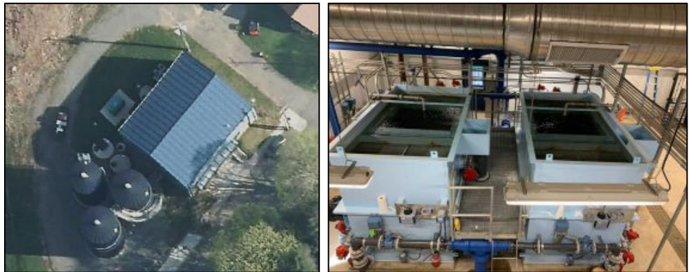
Figure 73. Structure with the maximum value ($8.9M) in floodplain of Marlinton (Marlinton Water Plant, Building ID: 38-08-0005-0088-0000_1002 )
