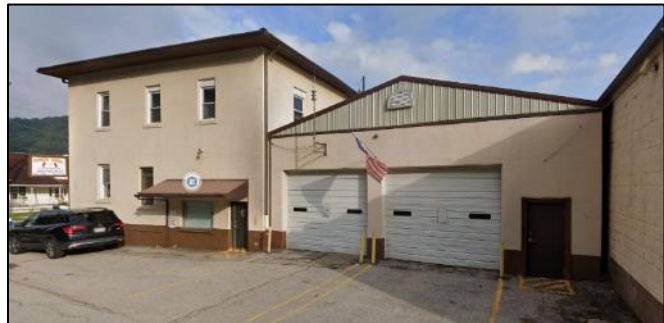
Figure 95. Clendenin Police Department (Building ID: 20-02-0007-0034-0000_103 )
