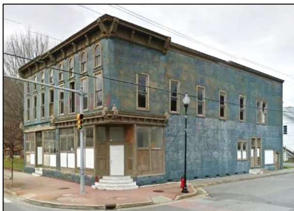
Figure 113. IOOF Lodge Building in Marlinton (Building ID: 38-08-0001-0021-0000_109 )
