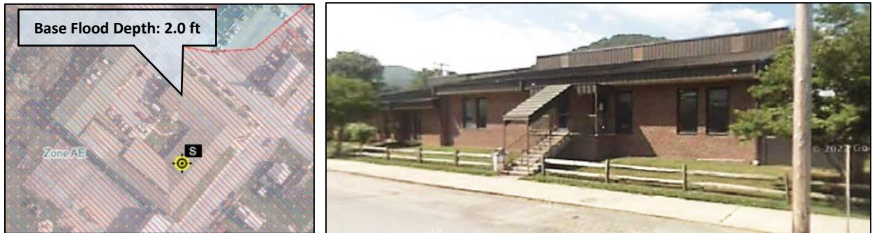
Figure 139. Highest estimated building loss in Marlinton ($248K), Marlinton Elementary School (Building ID: 38-08-0005-0009-0000_926 )
