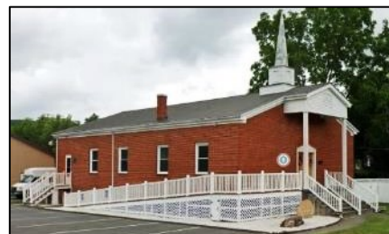
Figure 130. WSS Baptist Church in Floodway (Building ID: 13-17-0009-0073-0000 201 )
