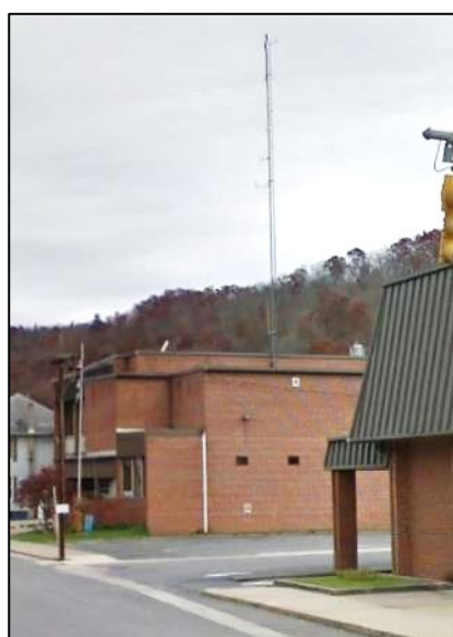
Figure 86. Marlington Police Department (Building ID: 38-08-0001-0096-0000_709A )
