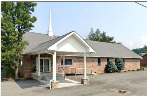
Figure 132. Greenbrier Ave. Church of God, Highest community asset value ($435K) in Rainelle’s floodplain (Building ID: 13-13-0005-0366-0000_373 )
