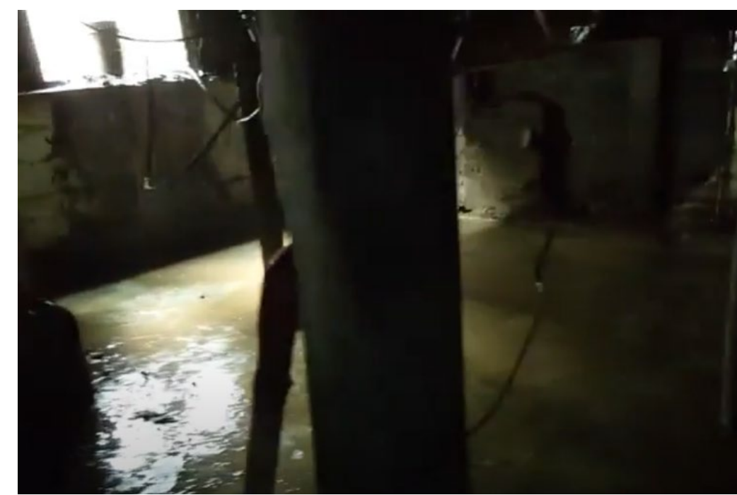
An inundated basement in the 2016 flood
