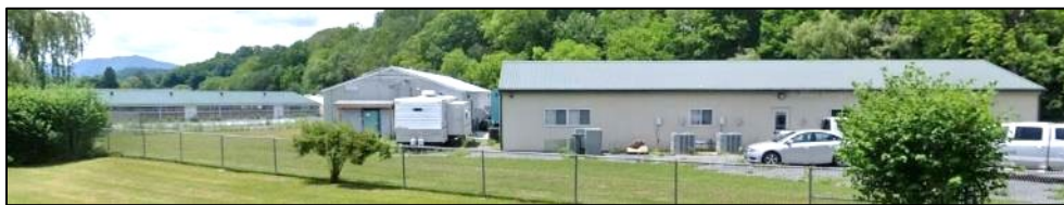
Figure 129. White Sulphur Springs National Fish Hatchery, Highest non-historical community asset value ($425K) and flood depth (2.4 ft) (Building ID: 13-17-0009-0206-0000 1087 )
