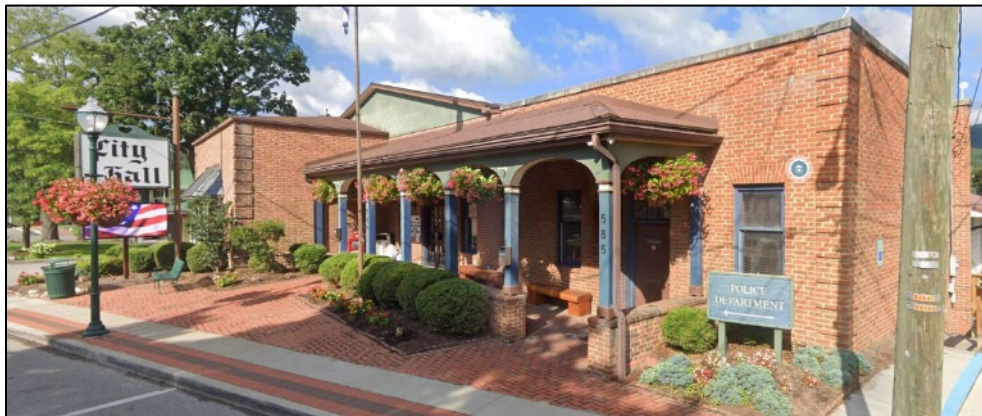
Figure 101. White Sulphur Springs Police Department (Building ID: 13-17-0011-0249-0000 585 )
