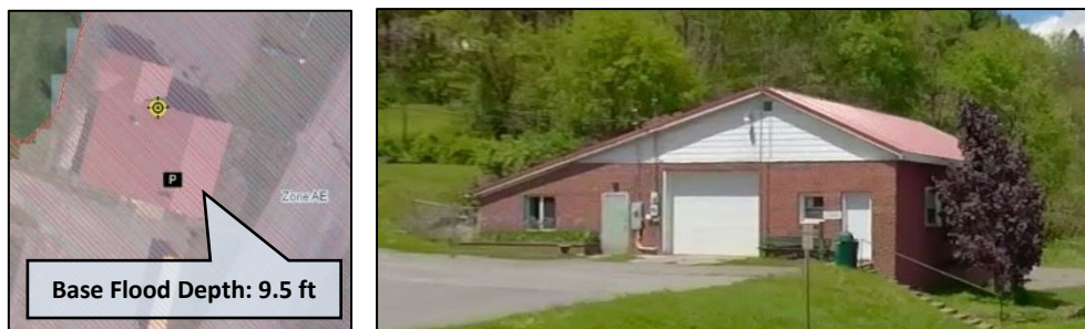
Figure 141. Highest estimated building loss in Camden-on-Gauley ($25K), Police Department, Storage Facility (Building ID: 51-01-0003-0094-0000_9676 )
