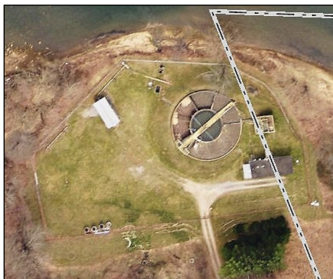
Figure 76. Structure with the maximum value ($880K) in floodplain of Richwood (City of Richwood Wastewater Treatment Plant, Building ID: 34-05-0030-0014-0000_408 )
