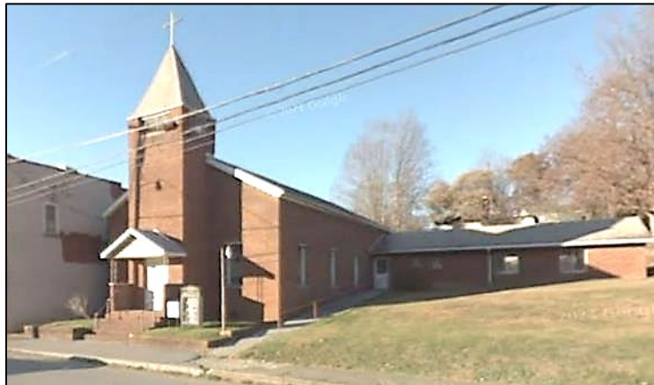
Figure 136. Bethel Methodist Church, in Camden-on-Gauley's floodplain (Building ID: 51-01-0003-0144-0000 9999 )
