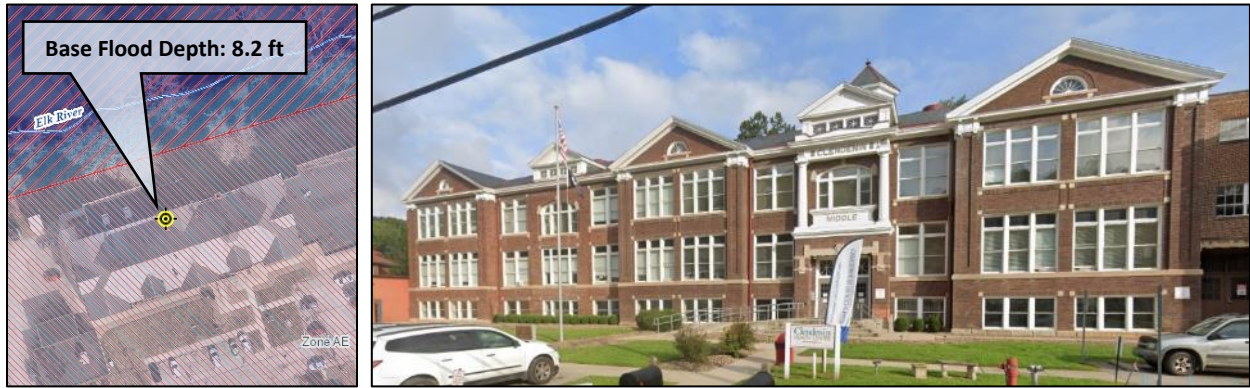
Figure 139. Highest estimated building loss in Clendenin ($84K), Clendenin Health Center (Building ID: 20-02-0007-0004-0003_107 )
