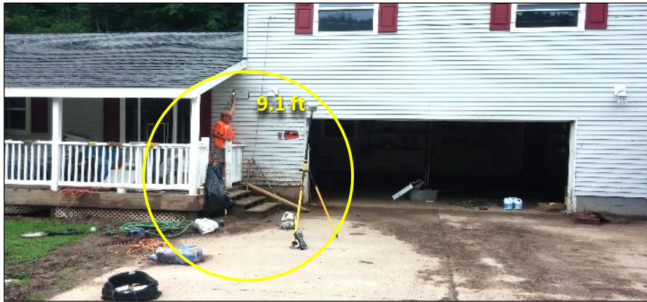
Figure 13. 2016 high-water mark in Camden-on-Gauley (9.1 ft) (Building ID: 51-04-0003-0006-0000_81 )
