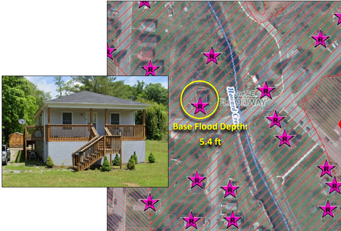
Figure 44. Structure with the maximum flood depth in White Sulphur Springs (Building ID: 13-17-0009-0009-0000_148 )
