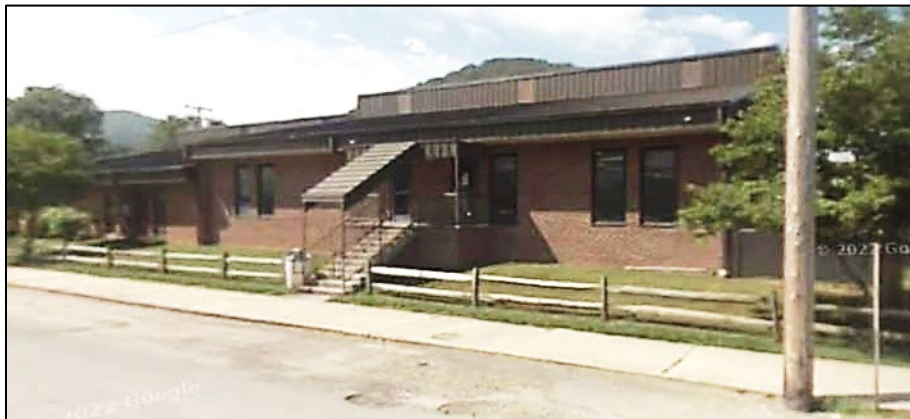
Figure 90. Marlinton Elementary School (Building ID: 38-08-0005-0009-0000_926 )
