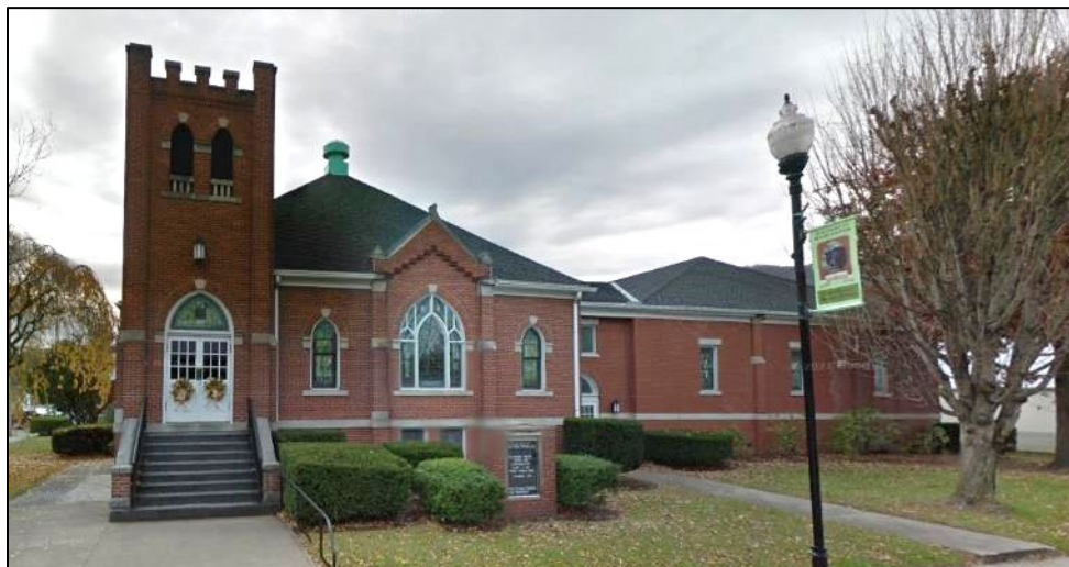
Figure 124. Marlinton Presbyterian Church in floodway (Building ID: 38-08-0002-0104-0000_815 )
