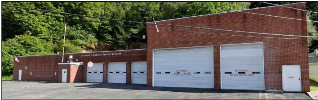
Figure 98. Rainelle Volunteer Fire Department (Building ID: 13-13-0005-0424-0000_212 )
