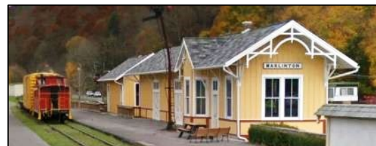
Figure 116. Marlinton Chesapeake & Ohio Railroad Station (Building ID: 38-08-0003-0041-0000_315 )
