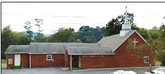
Figure 130. First Church of God in White Sulphur Springs' Floodway (Building ID: 13-17-0009-0066-0000 155 )
