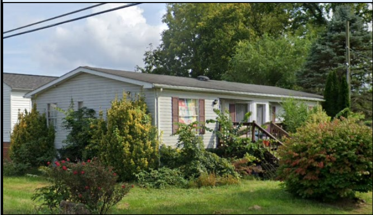
Double-wide Mobile Home in Ranson (FD: 2.2 ft) $33K; Year Built: 1993 (Post-FIRM) (Building ID: 19-08-0006-0019-0001_407 )
