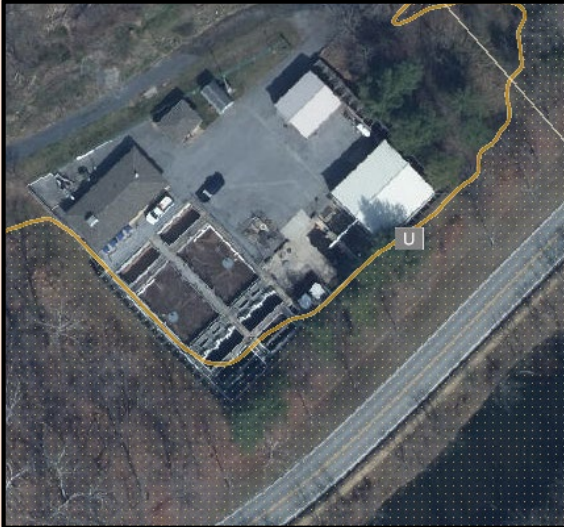
Harpers Ferry Bolivar PSD Wastewater Treatment Plant (FD: 1 ft) (Building ID: 19-05-0004-0025-0000_192 ) ($462K) Value source inflation adjusted to 2021
