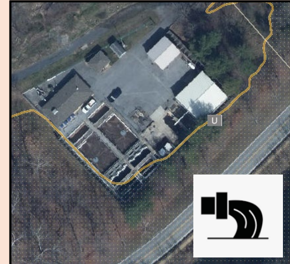
Harpers Ferry Bolivar PSD Wastewater Treatment Plant (FD: 1 ft) (Building ID: 19-05-0004-0025-0000_192 ) ($462K) Value source inflation adjusted to 2021
