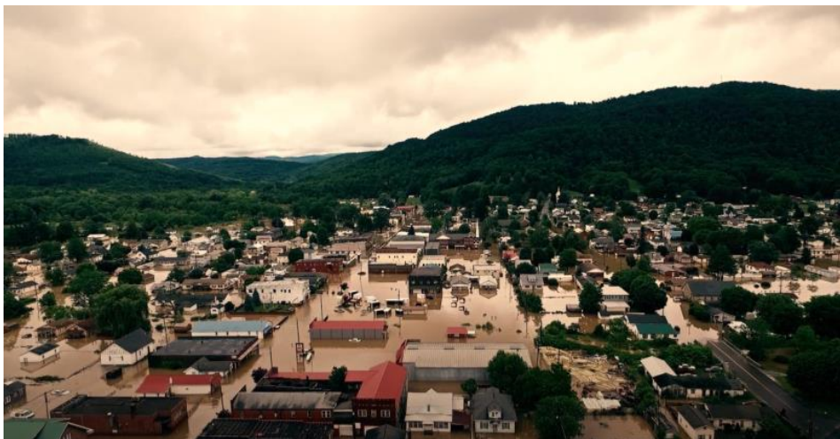
Rainelle, WV in Greenbrier County during the 2016 floods
