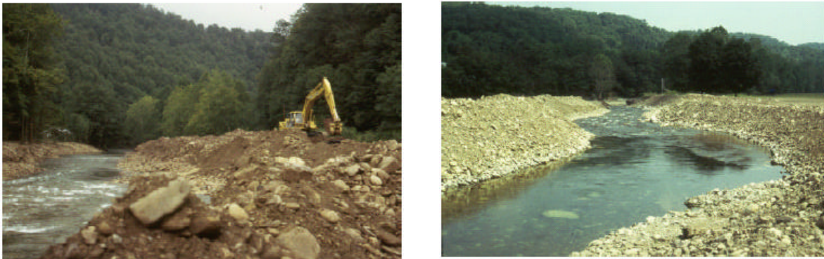
Figure H-3. Dredging of a small stream
