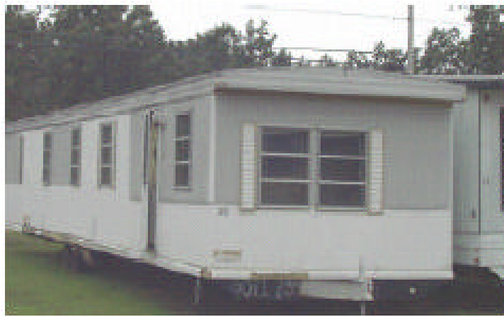
Figure A-1: Unsecured manufactured home
