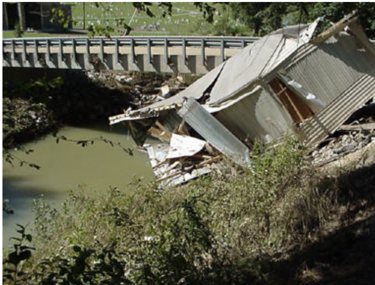
Figure E-1. Manufactured Home Blocking a Stream Crossing
