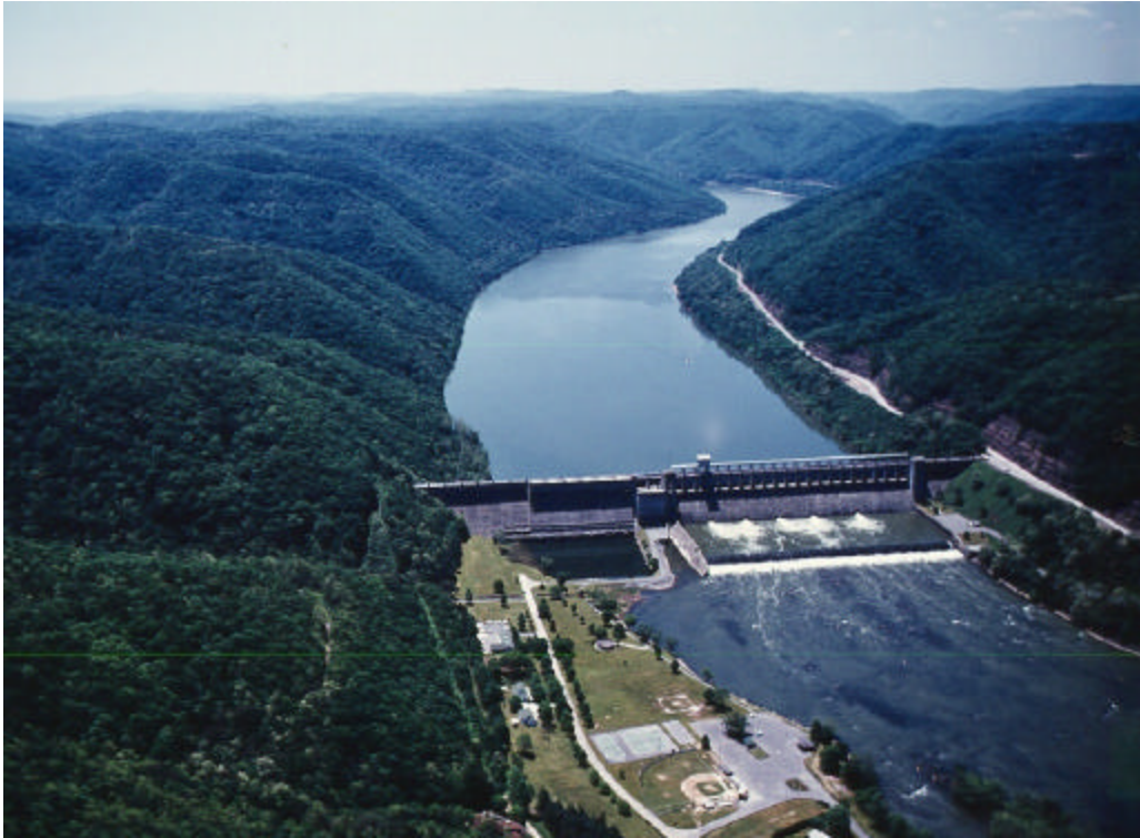
Figure L-4. Bluestone Dam and Lake, Hinton, WV
