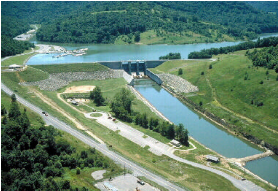
Figure 4-3 Burnsville Dam in Braxton County, West Virginia
