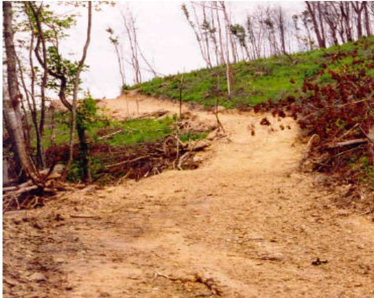
Figure F-5. Steep access road in timber removal area
