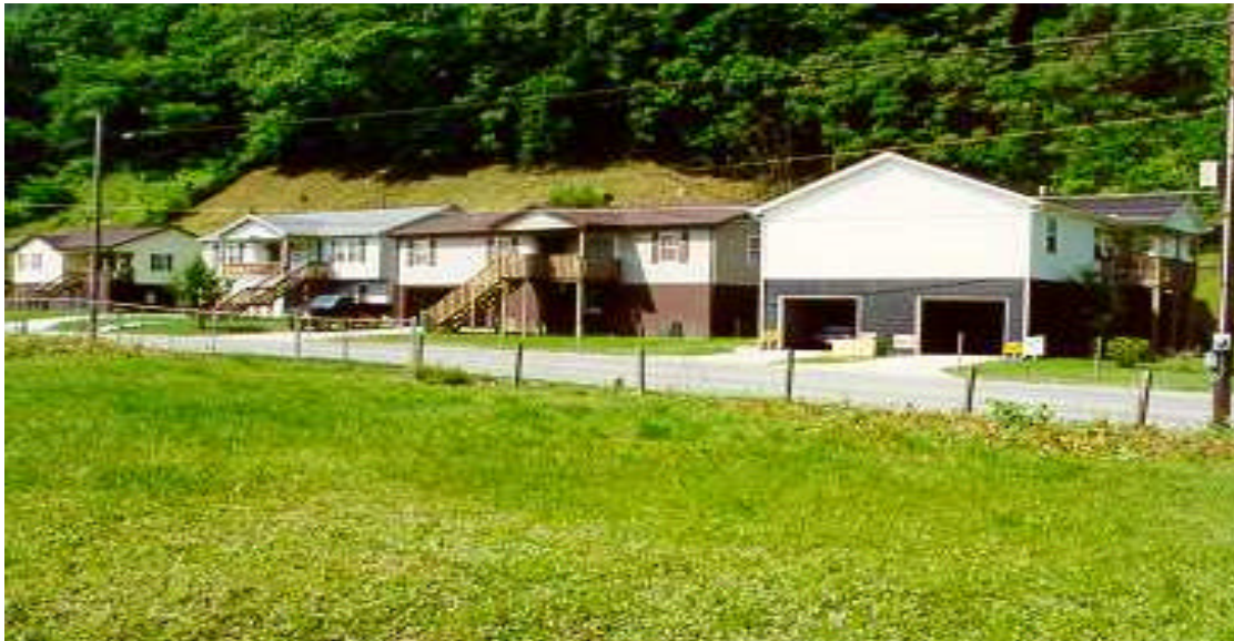
Figure L-8. Homes floodproofed on raised foundations
