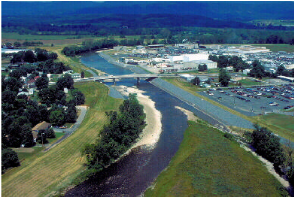
Figure No. 6 Levee project at Moorefield, WV
