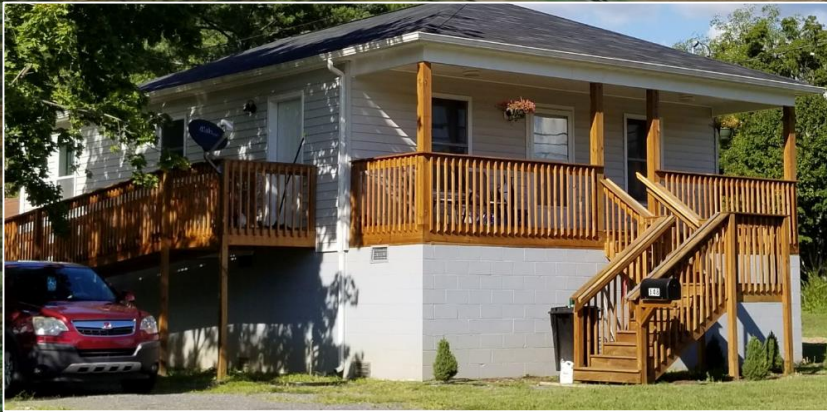
Elevated Structure (with flood vents)
