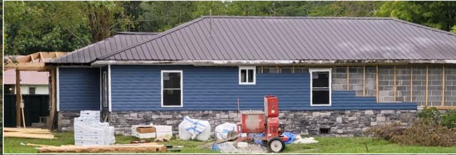
Substantially Damaged Structure Repaired
