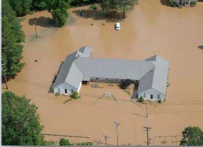
Flood Risk #1 WV Hazard
