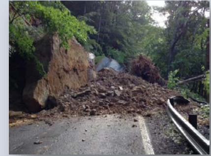
Landslide Risk #2 WV Hazard
