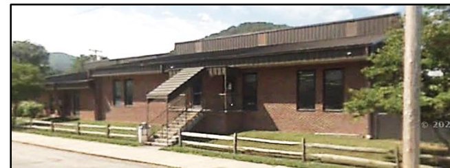
Marlinton Elementary School (Building ID: 38-08-0005-0009-0000_926 )
