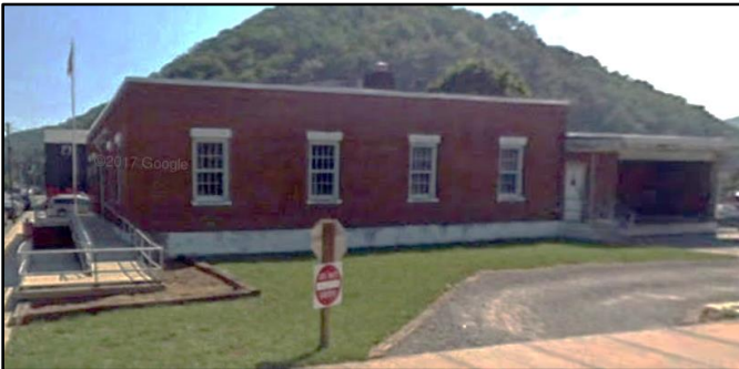
USPS in Marlinton Highest Non-Hist. CA Depth (4.8 ft) (Building ID: 38-08-0005-0006-0000_819 )
