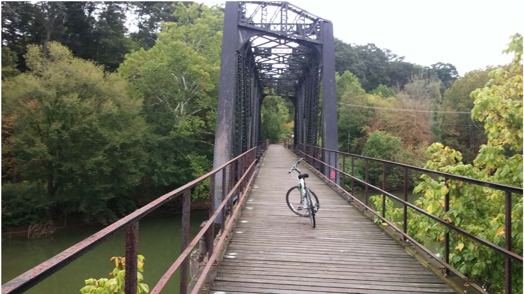
West Fork River Railroad Bridge, west of Fairmont, West Virginia
