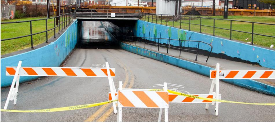
Figure 4: Localized flooding at railway underpasses impacts traffic movement in the City of Huntington. Photo credit: Sherry Wilkins, HSU
