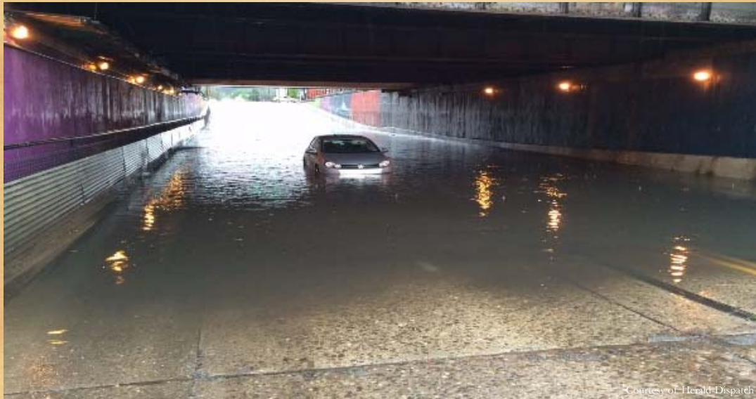
Courtesy of Herald-Dispatch
