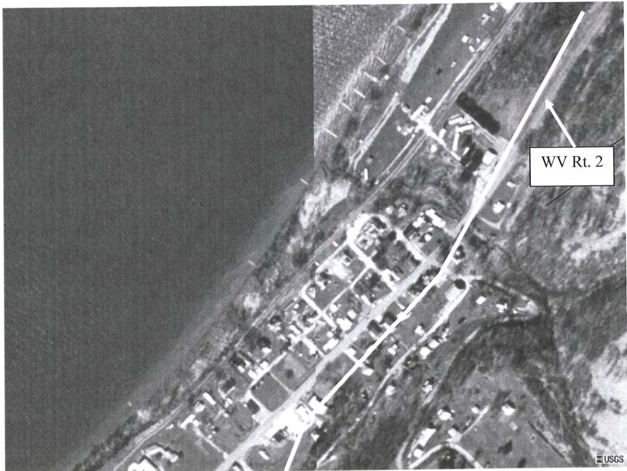
Plate 8. This plate shows the up river portion of Friendly. The white line denotes the extents of the 100-year flood boundary
