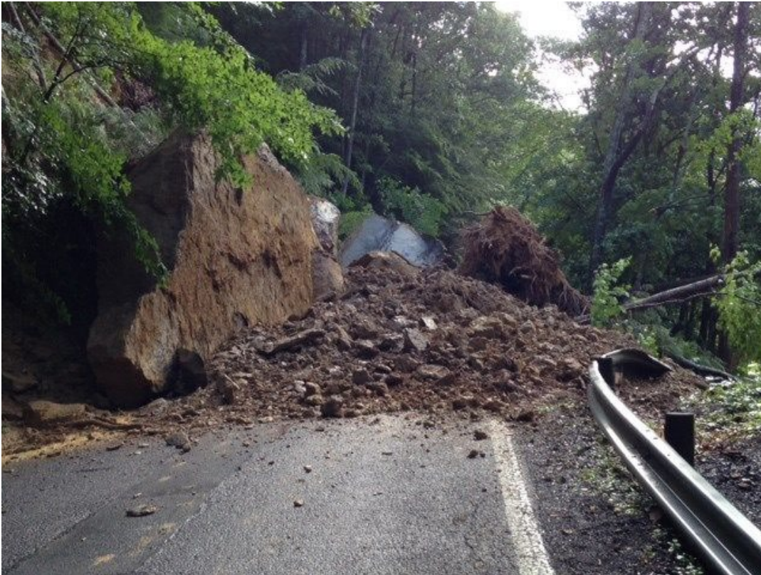
Landslide and rockslide across WV Route 82 (Photo by Collin Lawler, Channel 13 News, WOWK-TV) 75
