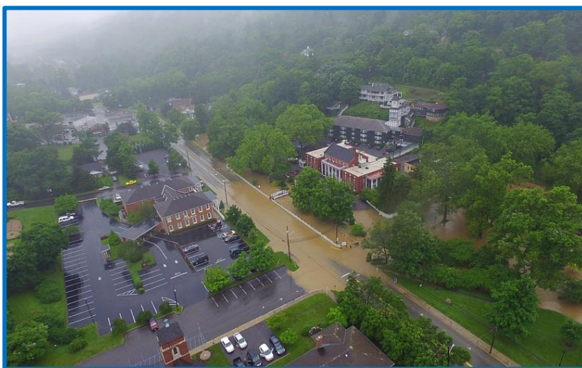
Figure 4.3.4-6: Town of Berkeley Springs, Morgan County during June 2018 flood event (Madison, 2018)
