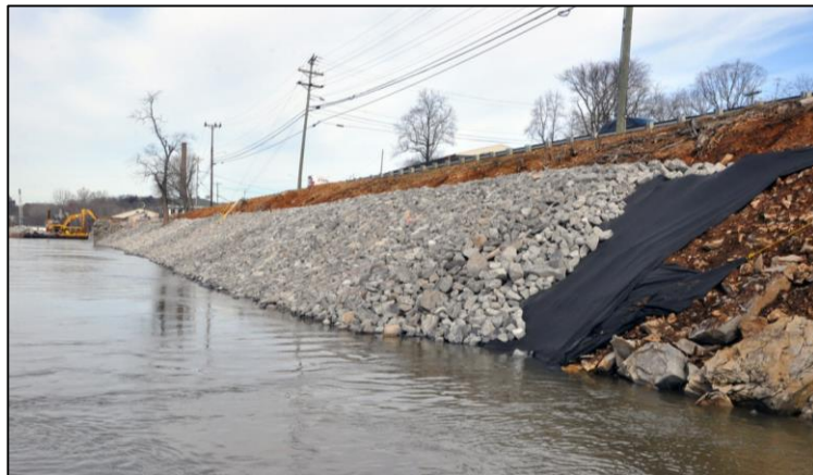
Reinforcing stream channels can help reduce erosion and landslide risk (photo by U.S. Army Corp of Engineers)
