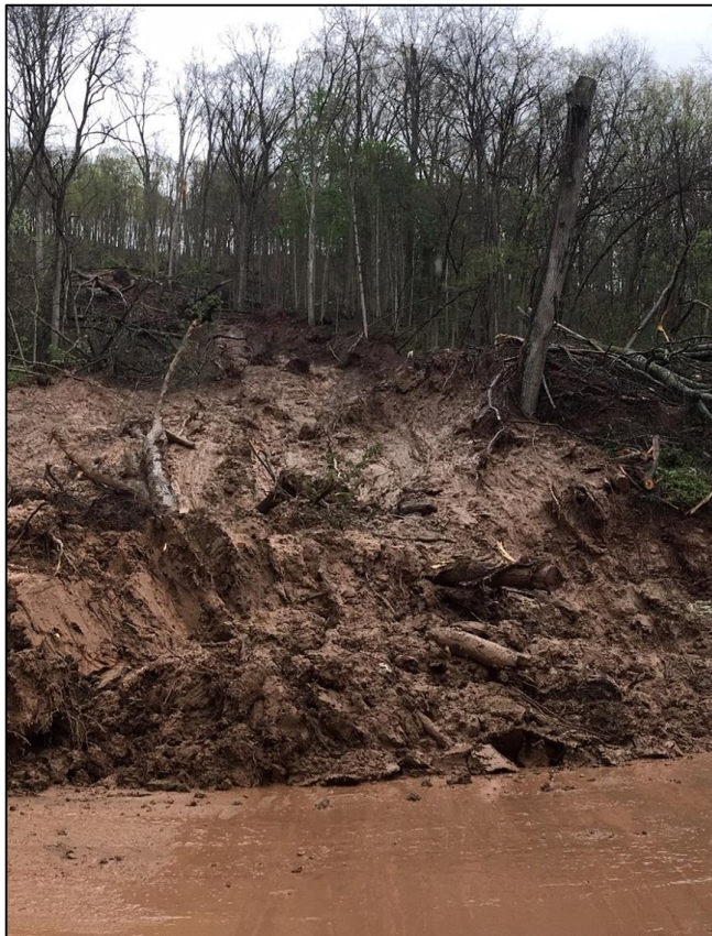
Water flowing over slopes can cause landslides (photo by WV Department of Transportation)
