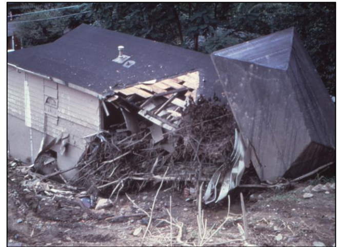
Landslides can cause extensive property damage (photo by J.S. Kite)
