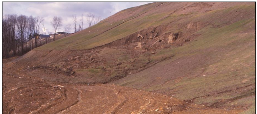
Excavating the base of slopes and removing vegetation can cause slope failure (photo by J.S. Kite)
