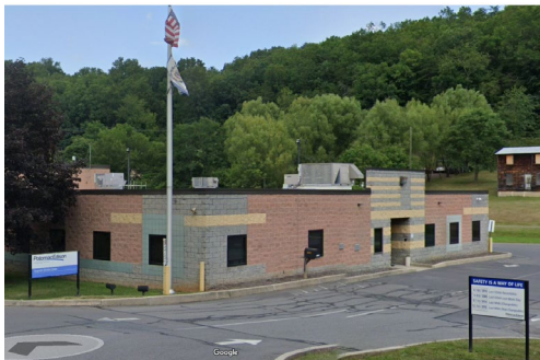
Potomac Edison Augusta Service Center Highest 2 nd Highest Non-Hist. CA Value ($1.4M) (Building ID: 14-05-0017-0024-0000_18444 )
