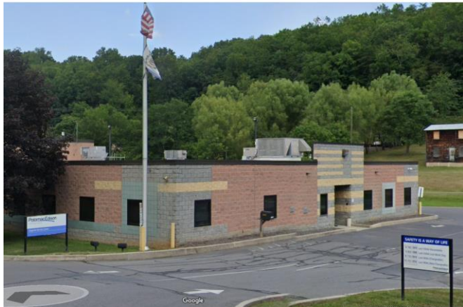
Potomac Edison Augusta Service Center 2 nd Highest Non-Hist. CA Value ($1.4M) (Building ID: 14-05-0017-0024-0000_18444 )
