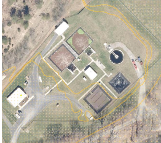
Central Hampshire Public Service District Wastewater Treatment Plant Highest Non-Hist. CA Value ($3.0M) (Building ID: 14-05-0018-0092-0000_251 )
