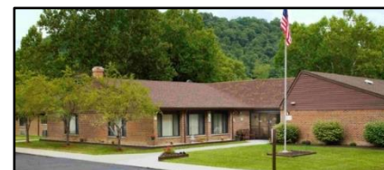
Pocahontas Center (Nursing Home) (Building ID: 38-08-0005-0065-0002_5 )
