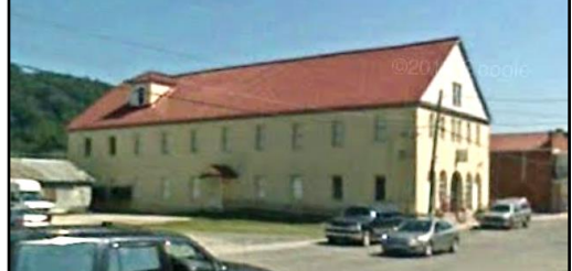
Marlinton Opera House Highest Hist. CA Depth (4.7 ft) & Value ($148K) (Building ID: 38-08-0002-0159-0000 818 )
