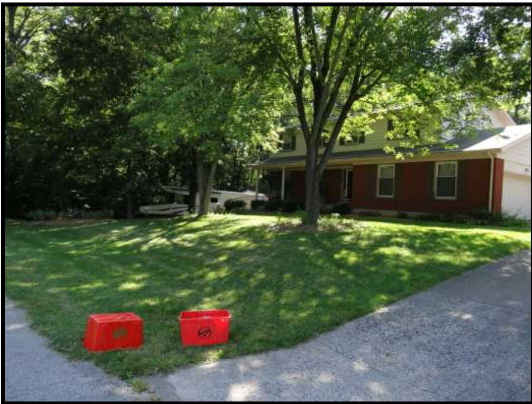
Photo 1 – View repetitive loss property from Seminole Drive, facing southeast. Portions of front yard have been built-up to prevent runoff from entering the house.
