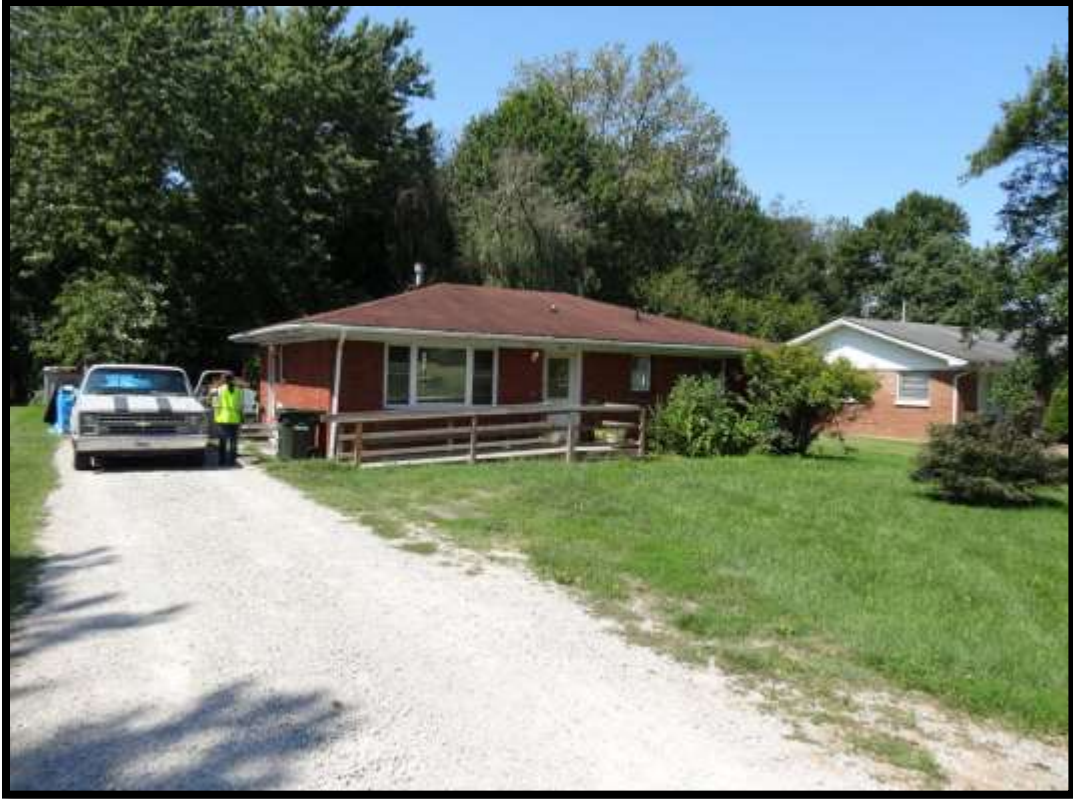
Photo 2: Center property considered to be in the repetitive loss area.
