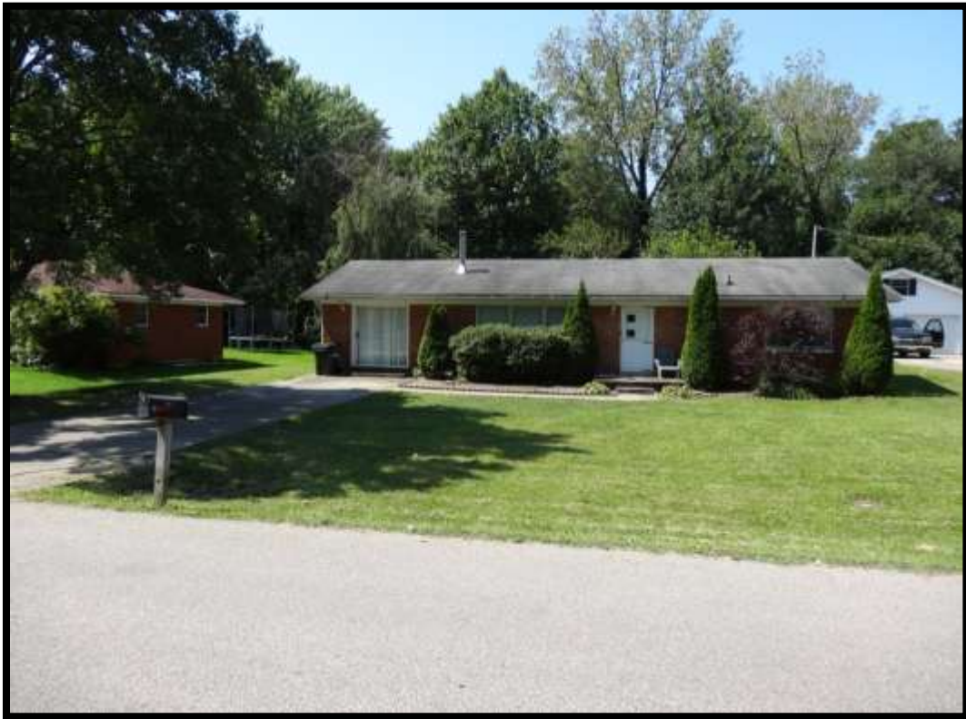
Photo 3: View of northern-most property considered to be in the repetitive loss area.
