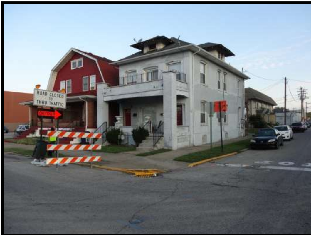
Photo 1 – View of property with historical flooding, viewed from the intersection of East Chestnut Street and Wall Street, facing northwest.
