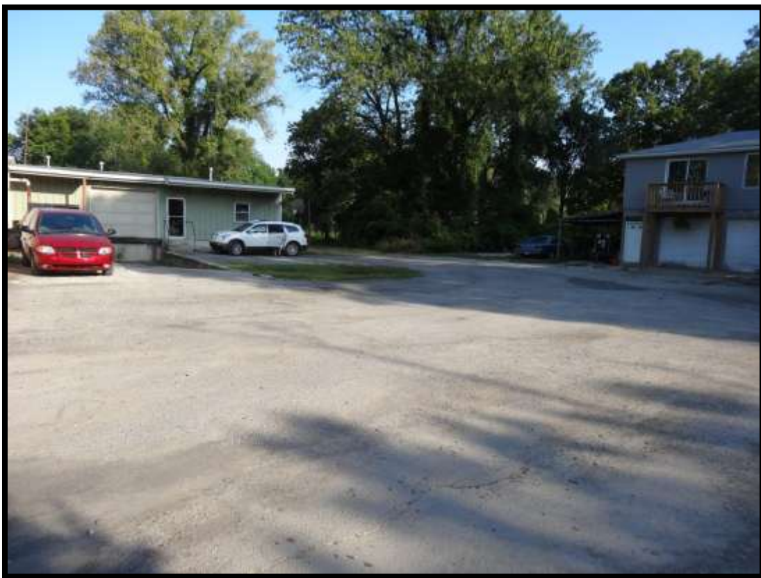
Photo 1 – View of westernmost property from entrance off of Hamburg Pike. Entrance road and parking lot were damaged by most recent flood according to local testimony.
