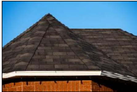
Asphalt Shingle Roof
