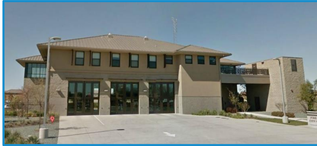
City of Sacramento Fire Station 43 (Natomas, CA)
