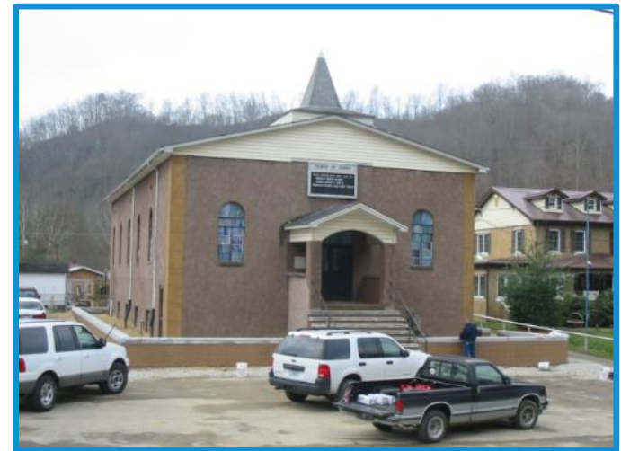
Masonry Wall (non-residential Crum, WV)
