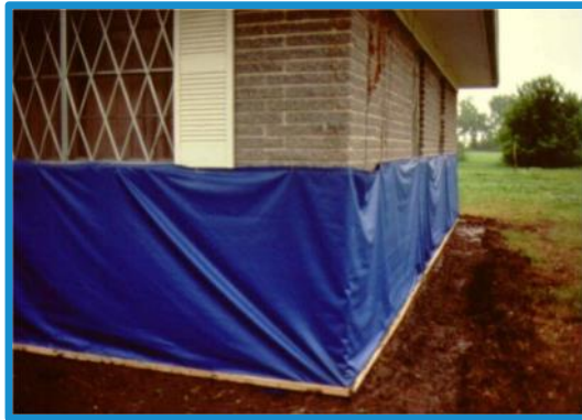
Dry Flood Proofing (Temporary)
