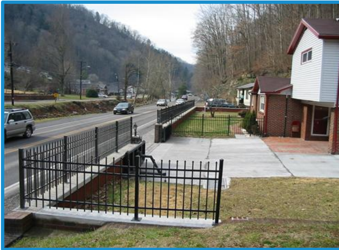
Masonry Wall (residential Grundy, VA)
