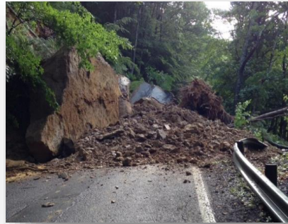
Landslide Risk #2 WV Hazard
