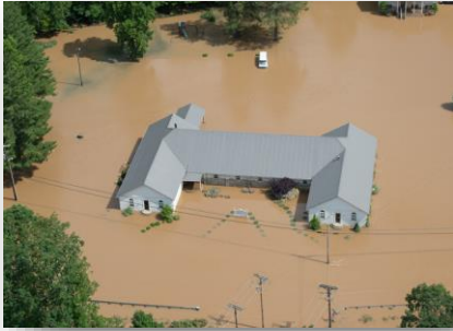
Flood Risk #1 WV Hazard
