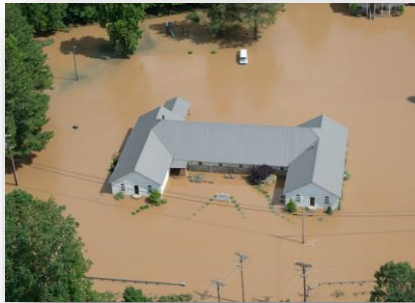
Flood Risk #1 WV Hazard
