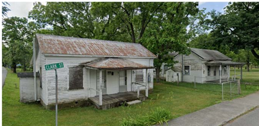
Figure 10: Examples of low valued (Red Tag) structures in Floodplain of White Sulphur Springs
