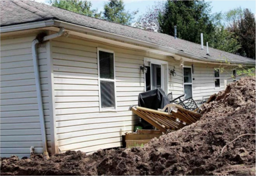
A landslide Sunday evening damaged a Washington Bottom home and forced the evacuation of several neighboring houses. (Photo by Michael Erb)
