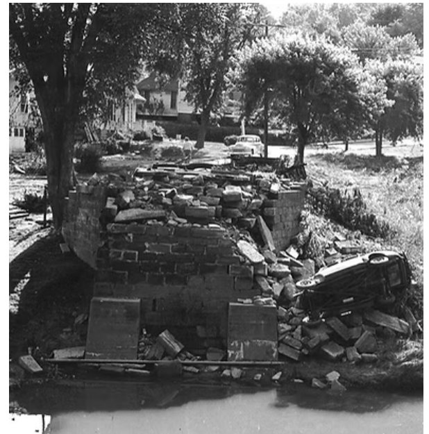
Foundation of Covered Bridge after the bridge washed downstream
