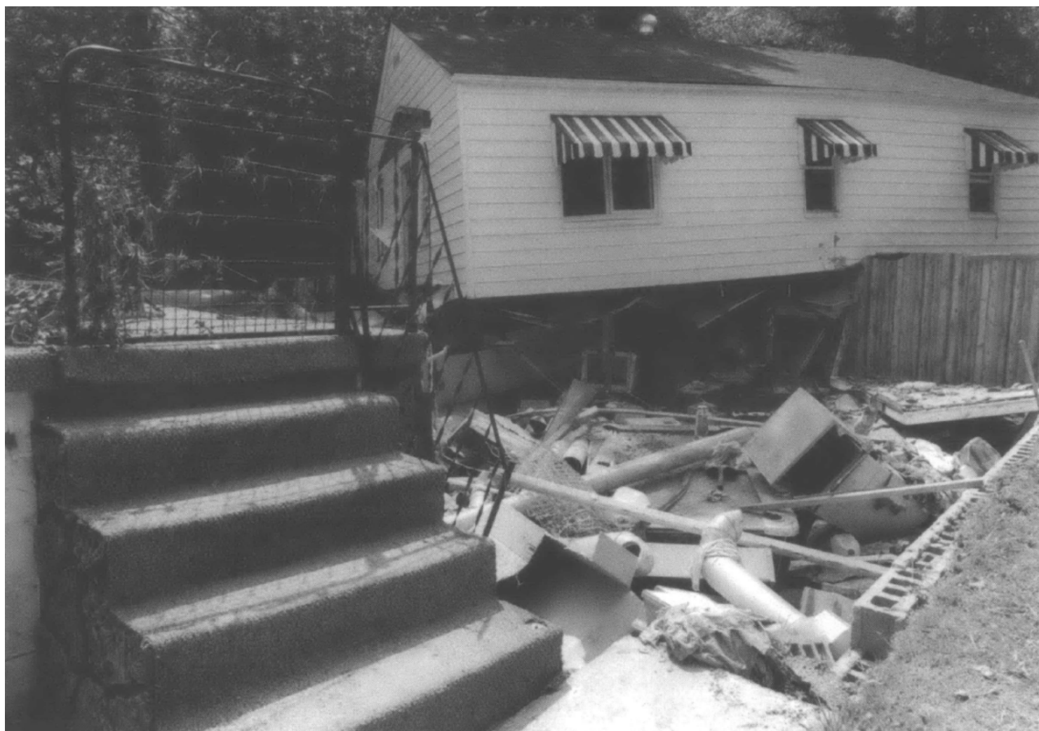
Steps to nowhere (Photograph by Bob Gates for Southern Exposure )
