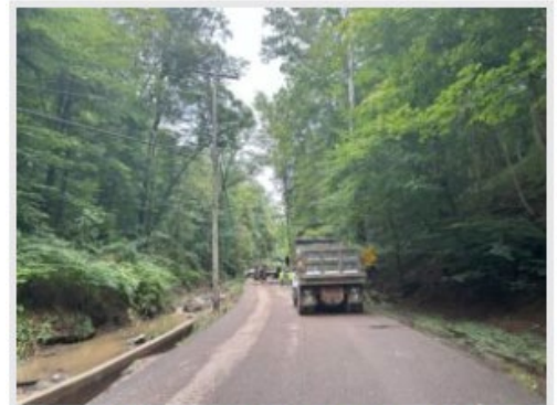
Crews working to remove debris along Garrison Ave. (Photo/Jack Carlson)
