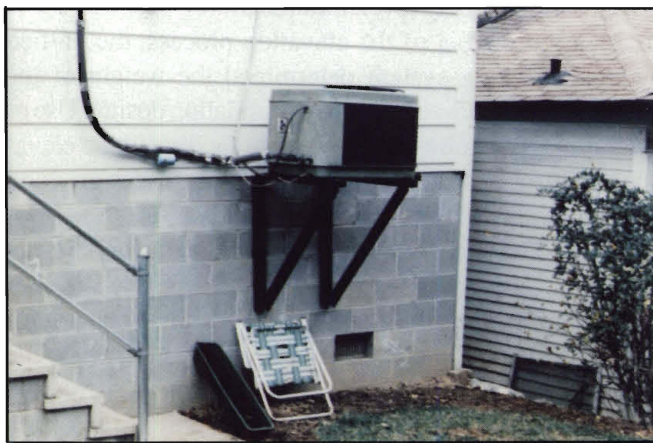
Figure 44.—Compressor Unit On Suspended Platform
