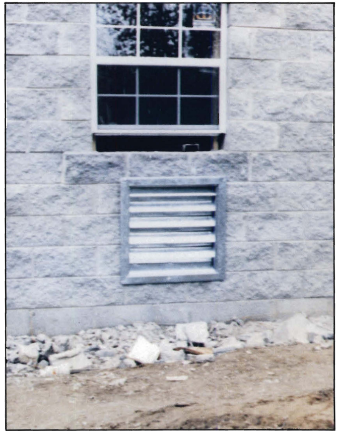
Figure 7.—Flood Louver Outside
