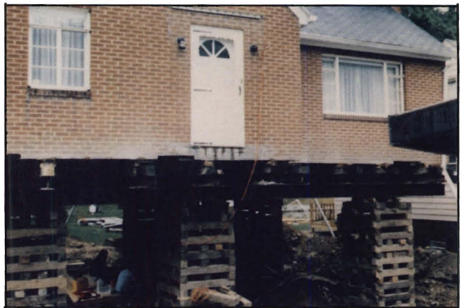
Figure 37.—Raised Structure On Cribbing
