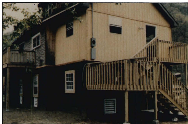
Figure 46.—Service Meter Relocated Onto Deck
