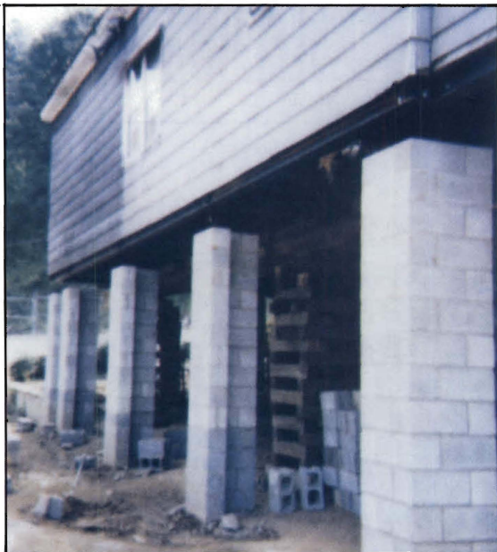
Figure 9.—House Elevated On Masonry Piers
