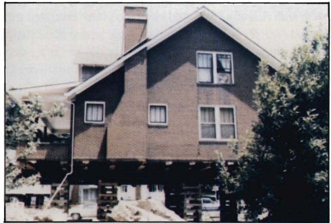
Figure 51.—Chimney Elevated With Structure
