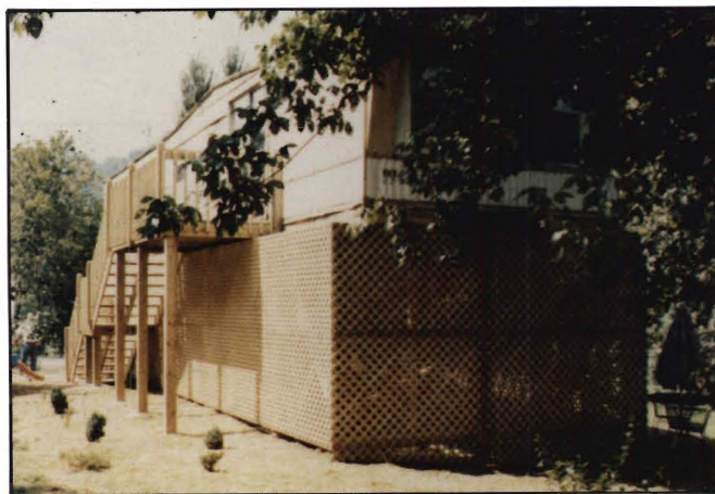
Figure 20.—Wood Post/Beam Lattice Panels
