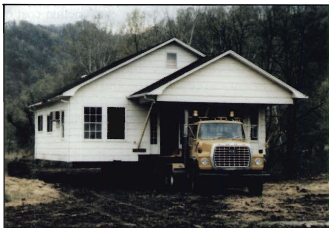
Figure 63.—Structure Being Relocated
