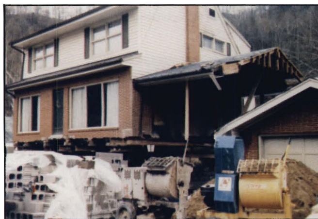
Figure 50.—Garage Separated Before House Elevation
