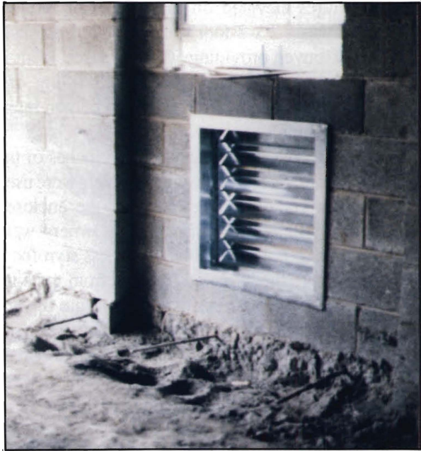
Figure 6.—Flood Louver Inside
