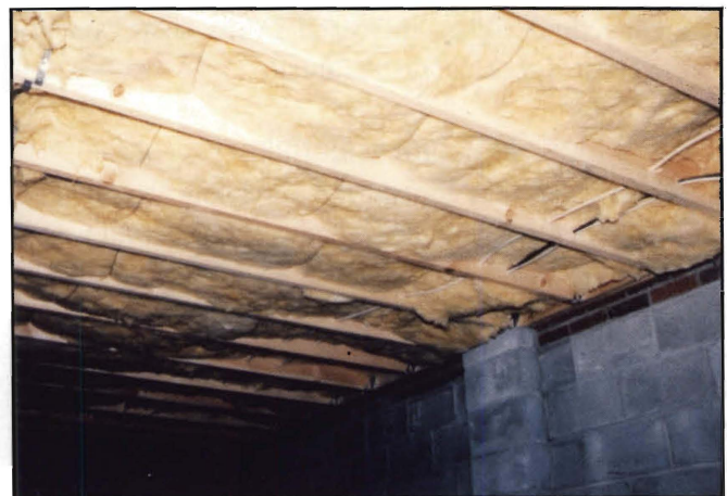
Figure 18.—First Floor Insulation
