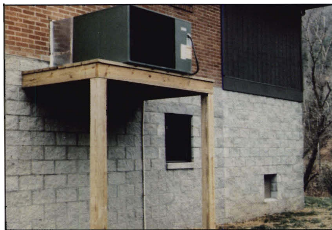
Figure 45.—Compressor Unit On Elevated Platform
