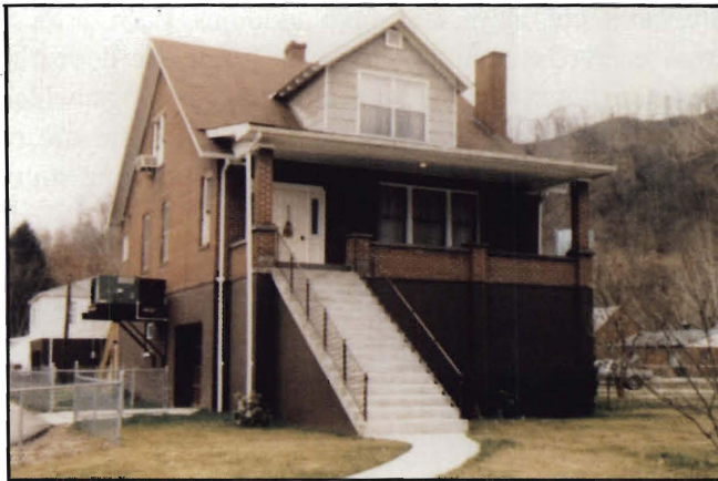
Figure 31.—Masonry Porch Raised With Steps
