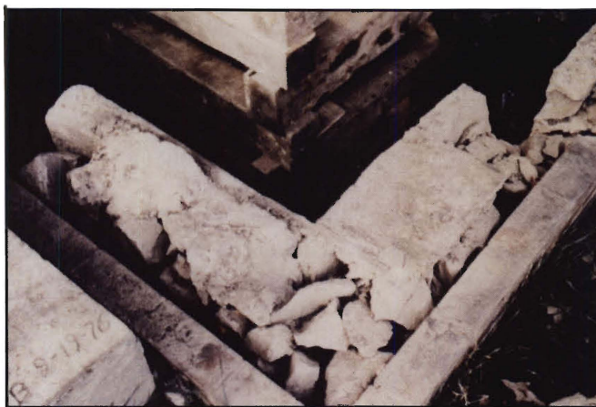
Figure 28.—Structure Damage Deteriorated Foundation
