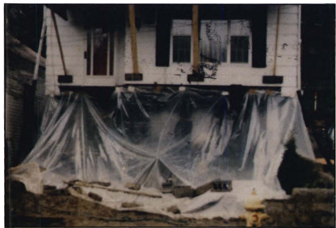
Figure 41.—Weather Protection Plastic Skirting
