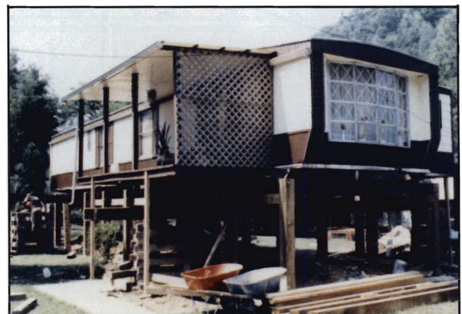
Figure 56.—Deck Raised With Manufactured Unit
