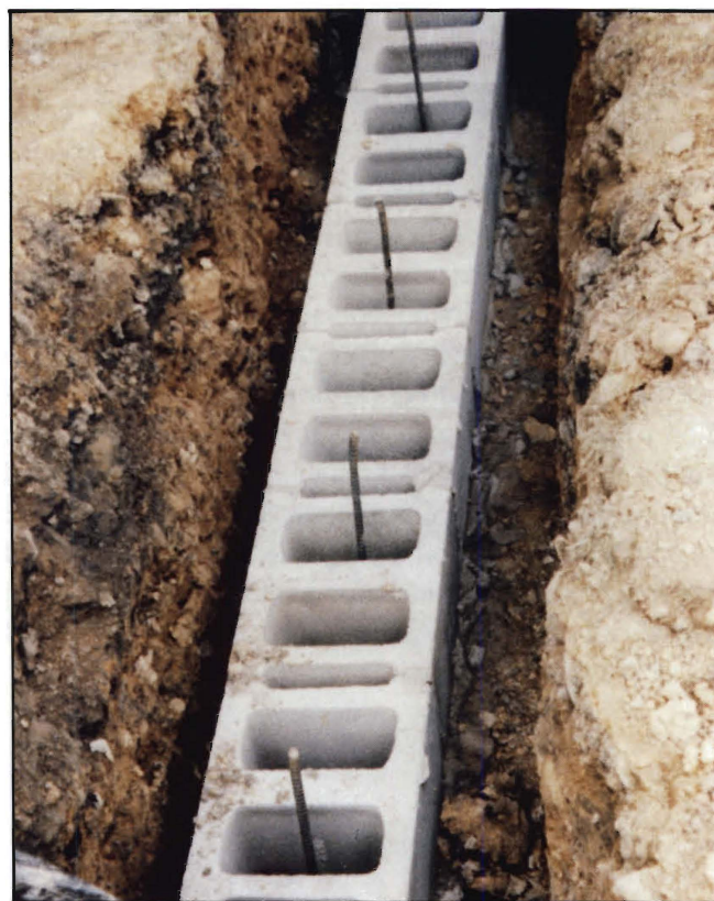
Figure 3.—Reinforced Masonry Wall Foundation
