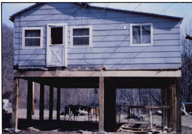
Figure 16.—Wood Post/Beam Post Spacing
