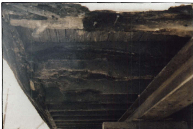
Figure 27.—Structure Damage Deteriorated Floors
