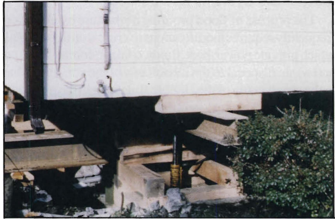
Figure 39.—Placement Of Hydraulic Jacks
