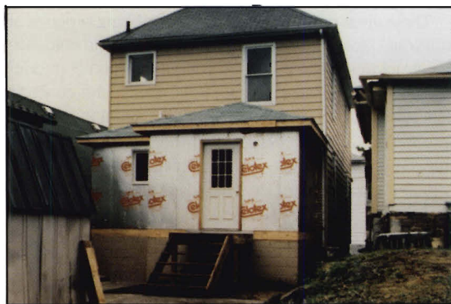
Figure 43.—Elevated Utility Room
