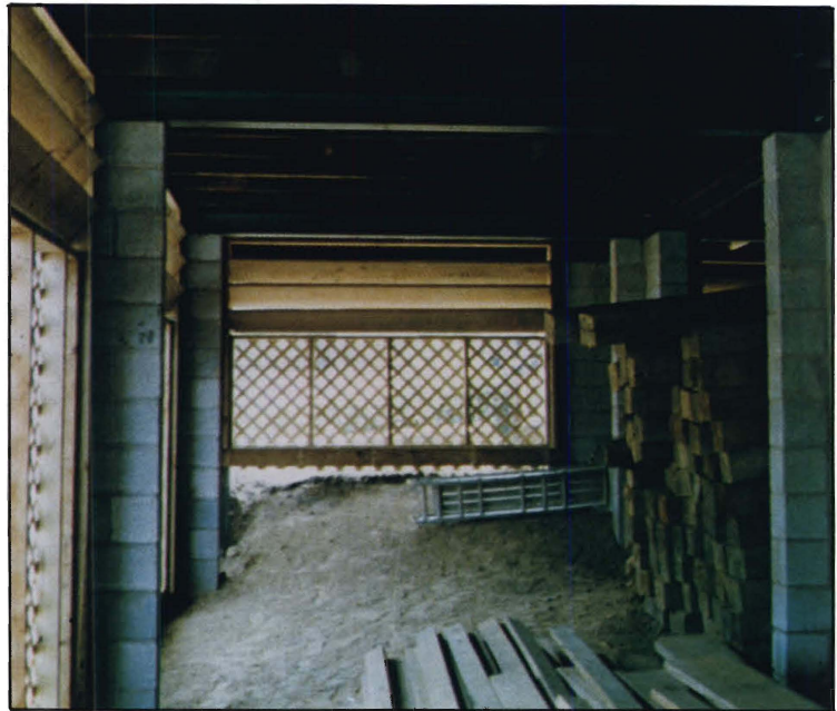
Figure 10.—House Elevated On Masonry Piers
