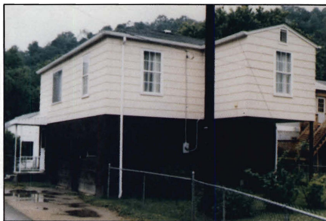
Figure 47.—Converted Garage Elevated
