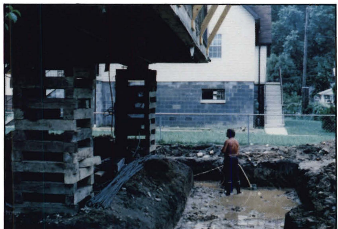
Figure 38.—Placement Of Cribbing Supports
