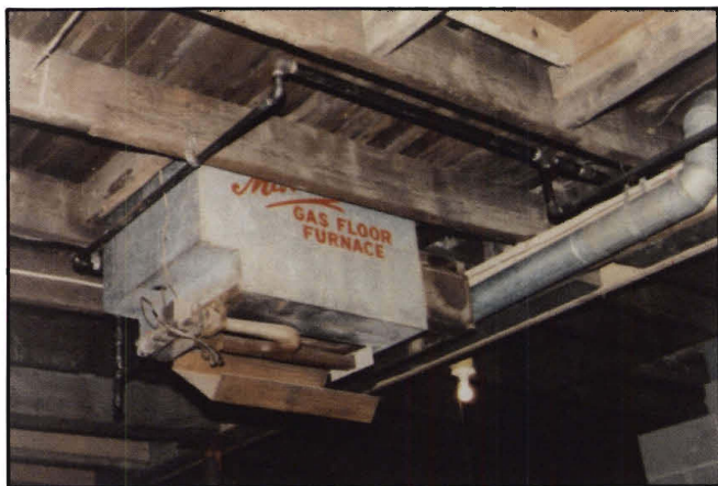
Figure 42.—Heating Unit Raised With Structure
