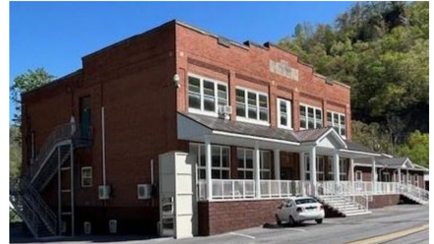
Elevated Town Hall / Police Station (Bradshaw)
