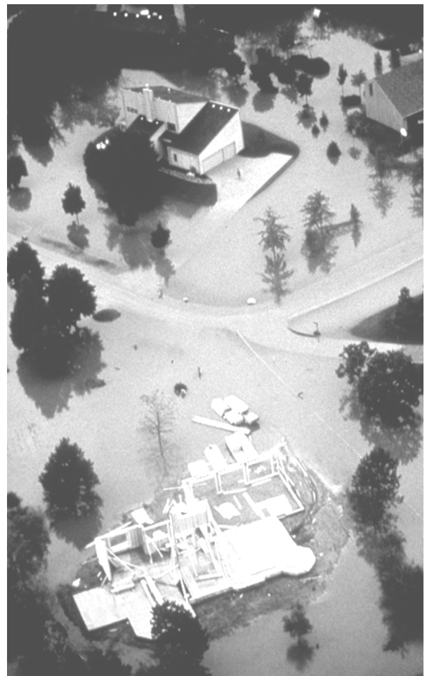
Figure 5-7. These two new buildings elevated on fill were not damaged by this 100-year flood.
