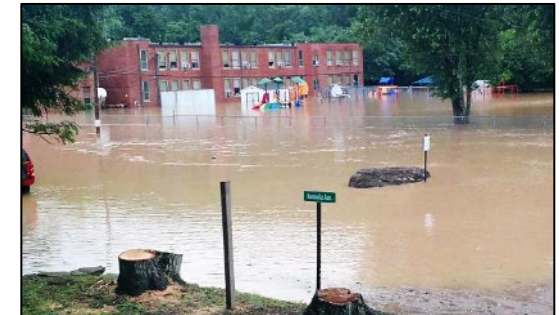
Clendenin Elementary School Kanawha County Inundated, Jun. 2016 (Demolished)
