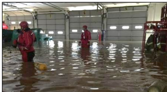
Clendenin Volunteer Fire Department Kanawha County Inundated, Jun. 2016 Building ID: 20-02-0007-0040-0000_109
