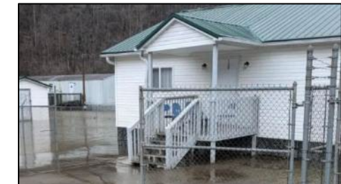
Cornerstone Church Matewan, Mingo County Inundated, Feb. 2025 Building ID: 30-08-0009-0071-0000_1028
