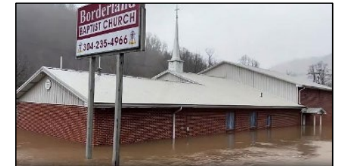
Borderland Baptist Church Mingo County Inundated, Feb. 2025 Building ID: 30-10-362K-0010-0000_46
