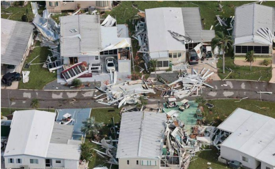
An aerial view of the damaged homes from Hurricane Ian seen in the vicinity of Fort Myers in September 2022. AL DIAZ adiaz@miamiherald.com
