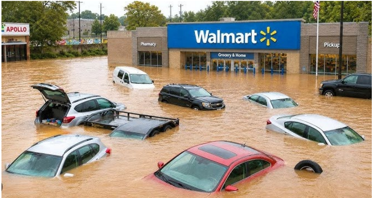
Figure 5. Multiple Submerged Vehicles (Weston Walmart), 22 July 2026 Flash Flood
