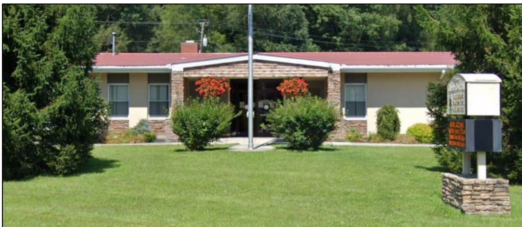
Figure 99. Rainelle Police Department (Building ID: 13-13-0004-0147-0000_1233 )
