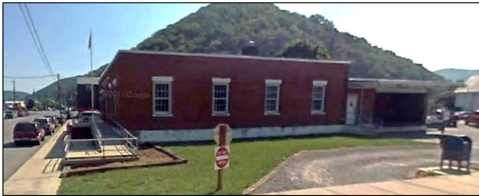
Figure 123. United States Postal Service (USPS) office, Highest non-historical community asset flood depth (4.8 ft) in Marlinton (Building ID: 38-08-0005-0006-0000_819 )
