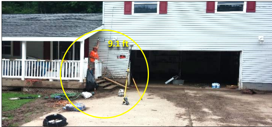
Figure 13. 2016 high-water mark in Camden-on-Gauley (9.1 ft) (Building ID: 51-04-0003-0006-0000_81 )
