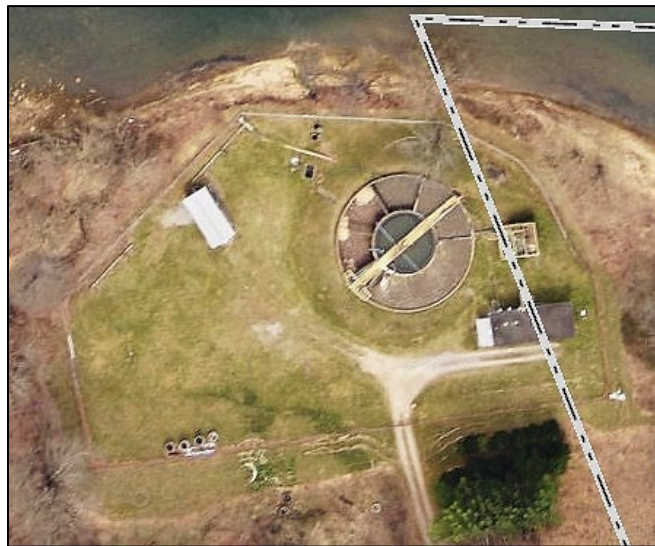
Figure 76. Structure with the maximum value ($880K) in floodplain of Richwood (City of Richwood Wastewater Treatment Plant, Building ID: 34-05-0030-0014-0000_408 )
