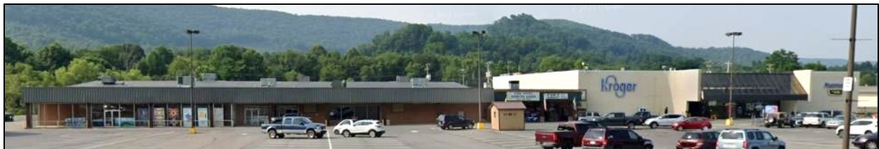
Figure 72. Structure with the maximum value ($1.49M) in floodplain of Rainelle (Building ID: 13-13-0004-0194-0000 506 )
