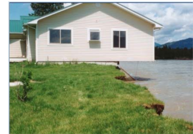
Clark Fork River, outside of Plains, Montana. Originally house was 30-40 feet from river bank and 1" above BFE
