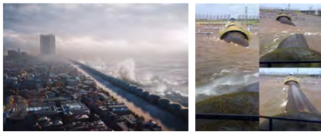
Figure 1a: Our visualisation of a pneumatic storm surge barrier positioned along the Rockaway Peninsula (NYC) and b the inflation of the Ramspl Bialgstuw between two lakes (clockwise image credit maritiemnieuws.nl)
