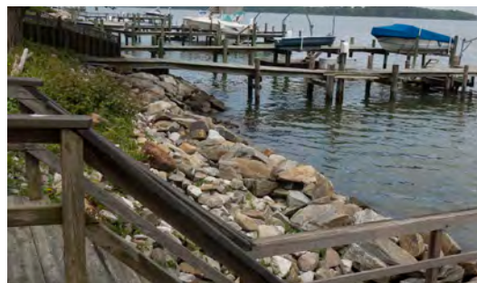
Riprap along a shoreline protects the property but can increase erosion at neighboring sites.
