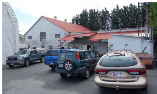
Many of the buildings associated with the Woodfield Fish and Oyster Company are susceptible to flooding.
