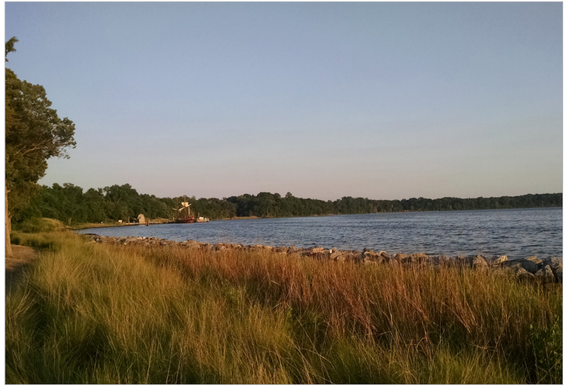
Figure 3.3 - Shoreline armoring and natural protection (rock in front of marsh) preventing erosion along the St. Mary's River to protect the bluffs where Historic St. Mary's City is located. St. Mary's City, St. Mary's County.
