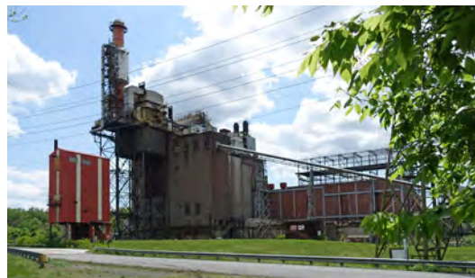
The abandoned power plant is located between the canal and the river.
