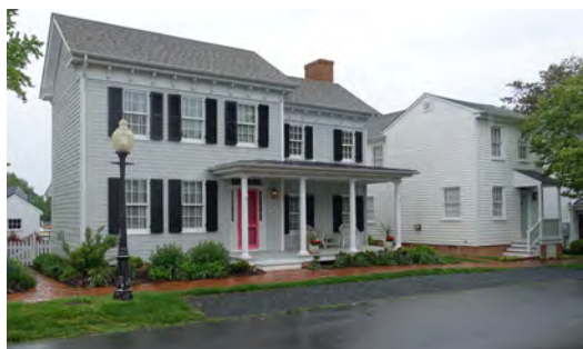
These two homes were recently elevated. The entrance stair for the home on the right was modified.
