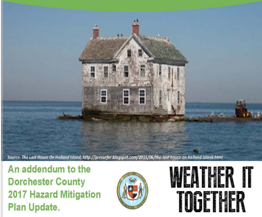
Figure 2.35 - Dorchester County addresses historic and cultural resources in a 2018 addendum to their 2017 Hazard Mitigation Plan Update.
