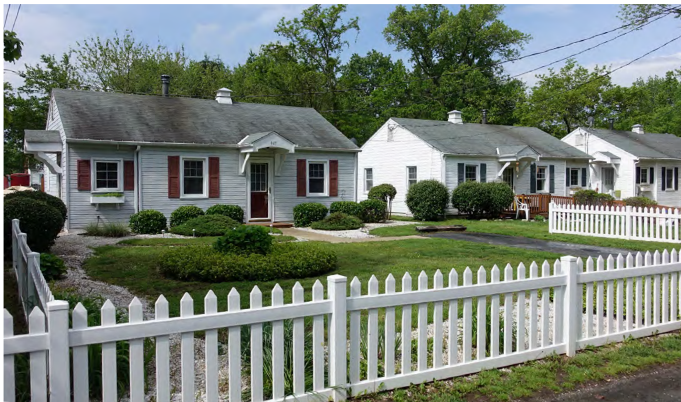
In 1996 indoor plumbing was installed in Galesville, including these homes on West Benning Road, improving the quality of life for its residents.
