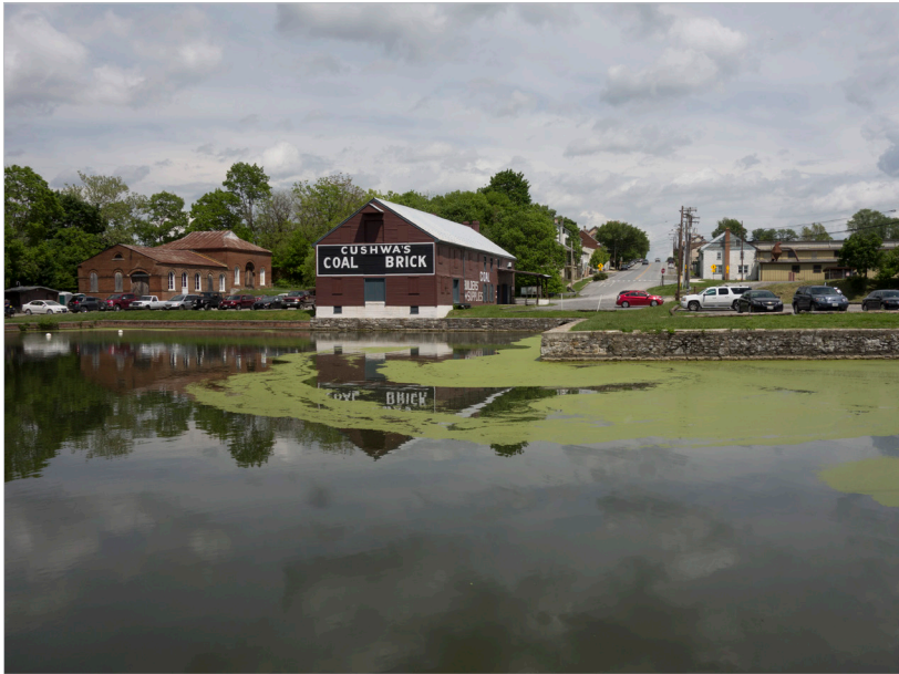
Figure 2.37 - Acceptance of building flooding: the earliest portion of this building, originally a warehouse, dates to the turn of the 19th century. The building was adapted to be a visitor center despite the risk of flooding. Flood openings are visible beneath the unpainted brick along the river-facing façade. Williamsport, Washington County.
