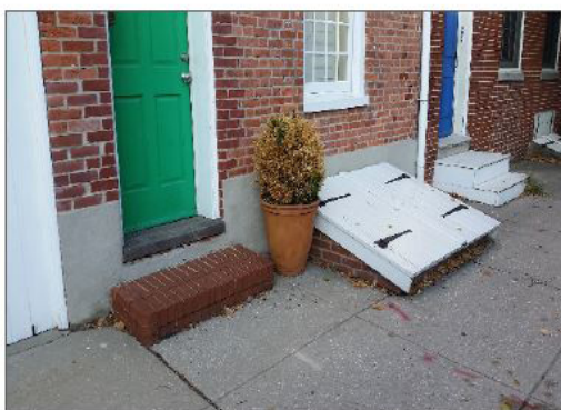
2. Foundation wall and basement access (Front)
