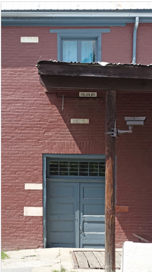
Figure 2.14 - Chesapeake & Ohio Canal Cushwa Warehouse (constructed circa 1790 – 1810) located at the canal’s edge has historical high watermarks visible in white block on the face of the building noting the depth of flooding from five food events from the mid-19th to early-20th century. Williamsport, Washington County.
