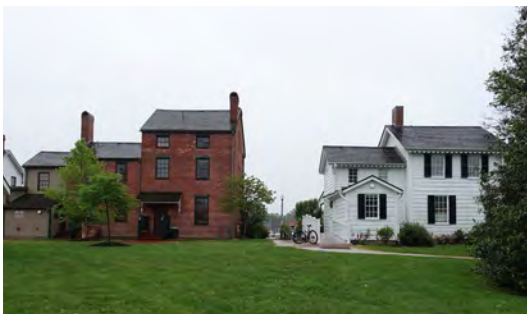
Several buildings associated with the Maritime Museum have been elevated, including the brick buildings to the left.
