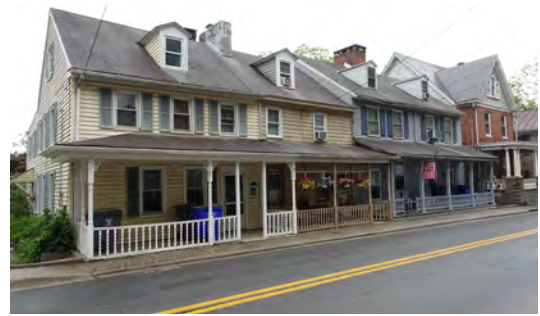
A handful of homes were constructed with the first floor level at about the same elevation as the sidewalk.
