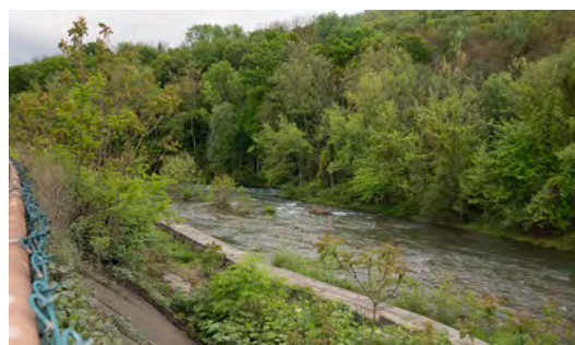
A concrete levee is located along Georges Creek approaching the North Branch of the Potomac.
