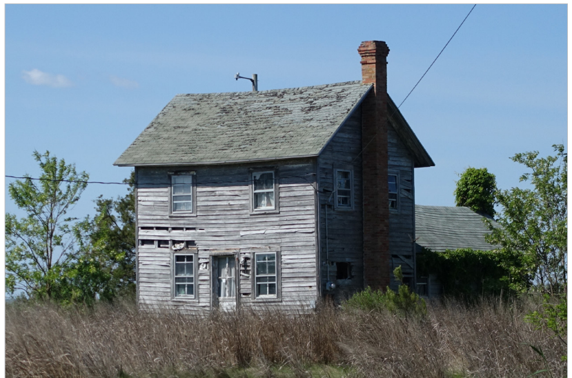
Figure 2.39 - Abandoned historic home on Hooper's Island, Dorchester County.
