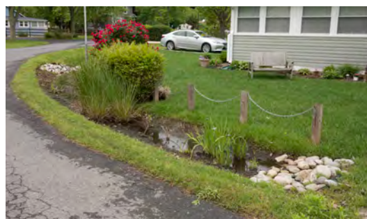
Rain gardens have been installed in Columbia Beach.
