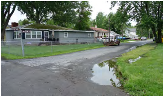
The cottages in Columbia Beach are generally one-story, wood framed buildings.
