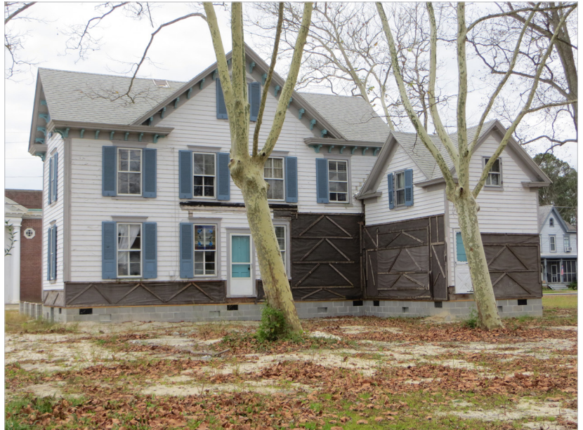
Figure 3.18 - Flood openings are barely visible within the elevated concrete block foundation along the second course of blocks just above the ground level, minimizing their impact on the house's character. The darker, higher openings are crawlspace vents. Crisfield, Somerset County.
