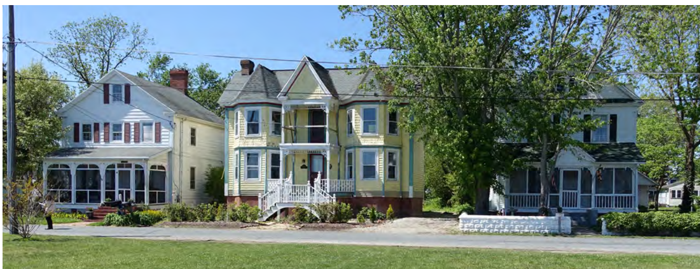
The elevation of the central residence altered the relationship between the porch and the street and required modification of the entrance stair. Also note the concrete foundation has been tinted a brick color.
