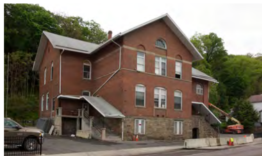
The Catholic school, now abandoned, was a focal point of the community. The school was demolished after the site visit.
