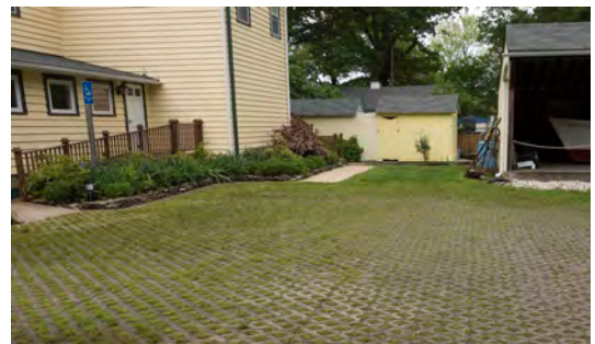
Permeable paving facilitates storm water absorption into the soil.
