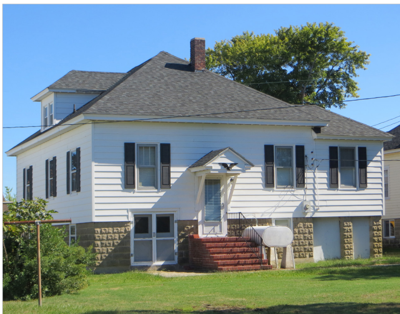
Figure 2.34 - House constructed on a higher foundation in the 1930s after an unnamed coastal storm. Ewell, Smith Island, Somerset County.
