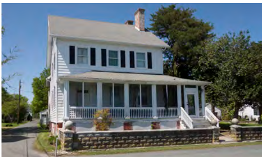
A small opening is located in the rusticated block wall, potentially restricting site drainage.
