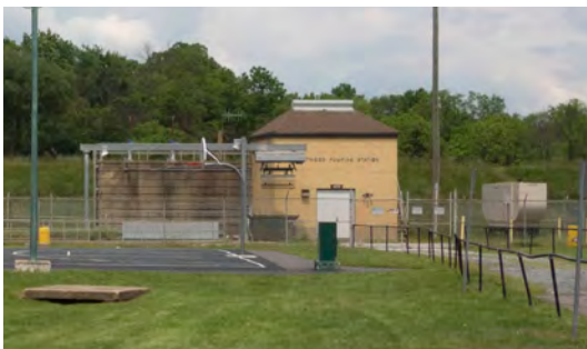
The Bladensburg Pump Station is located at the base of the levee adjacent to the basketball court.
