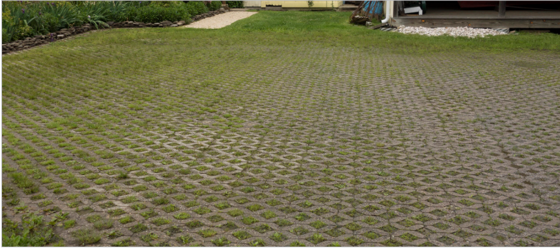
Figure 3.9 - Zoning requirements can include limiting stormwater run-off through the use of pervious paving. Shadyside, Anne Arundel County.
