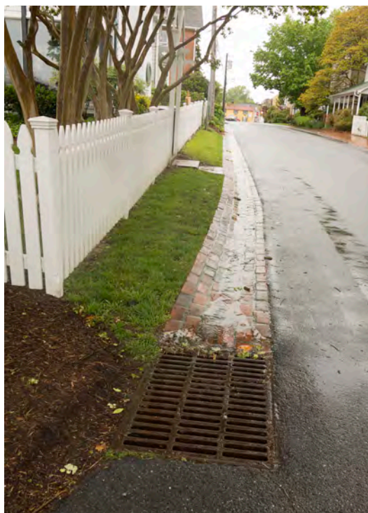
Storm water drainage is gravity-fed along the street edge to a storm drain.
