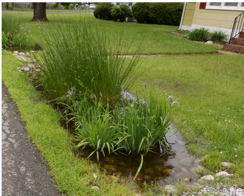
Figure 2.32 - Rain gardens provide an efficient means of minimizing stormwater runoff and can often be integrated into existing landscaping. Shady Side, Anne Arundel County.
