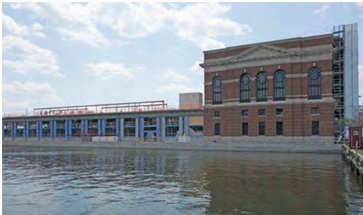
The former Fells Point Recreation Pier is being redeveloped as a hotel.
