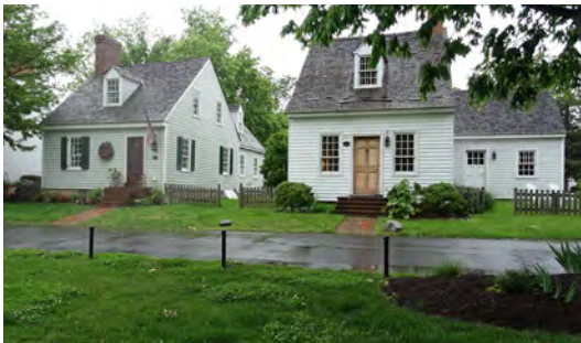
Several of the small wood-framed workers homes have been relocated onsite, away from the street.
