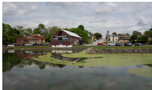
The NPS currently occupies the Cushwa building, and have located sensitive equipment on the 2nd floor.
