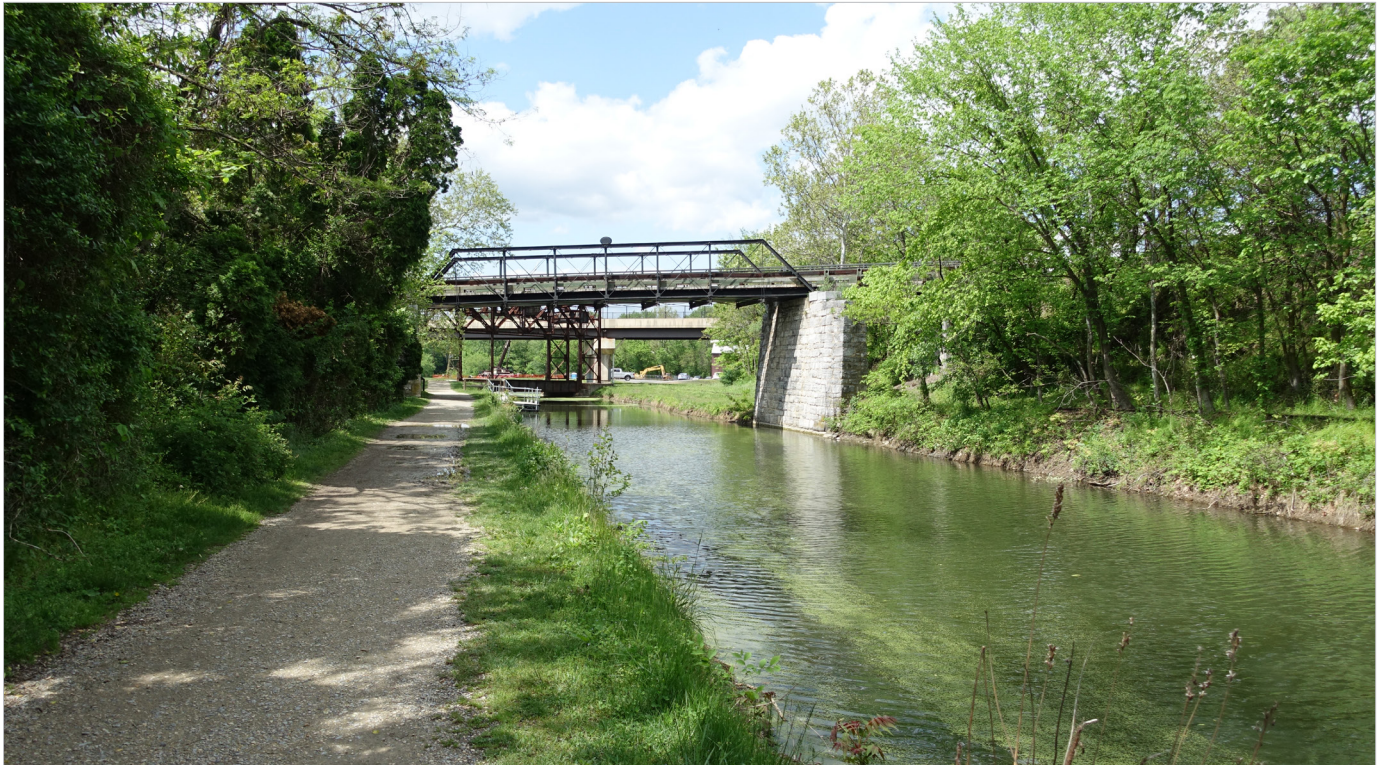
Figure 2.26 - A pedestrian path with pervious paving provides a recreational amenity for the community while facilitating stormwater absorption in the event of a flood. Williamsport, Washington County.
