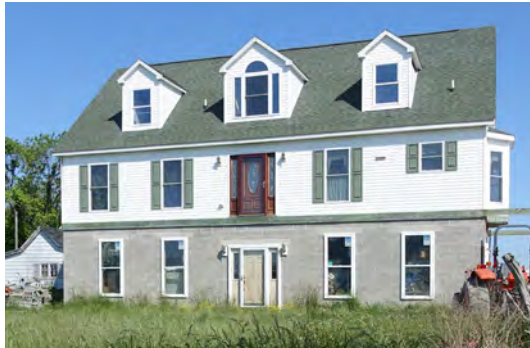
This home on Hoopers Island was elevated a full story and includes a new concrete block lower level.
