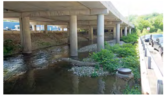
The waterway is highly restricted and prone to flooding in a minor rain event.
