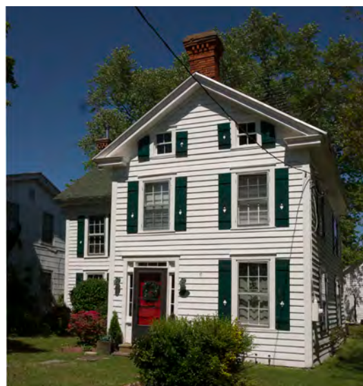
The first floor of this residence is close to grade, and it has suffered repeated damage from flooding.
