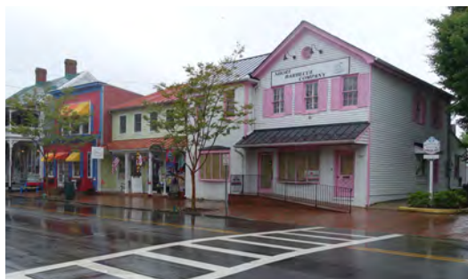
Elevating commercial buildings presents accessibility challenges and may require installation of a ramp.
