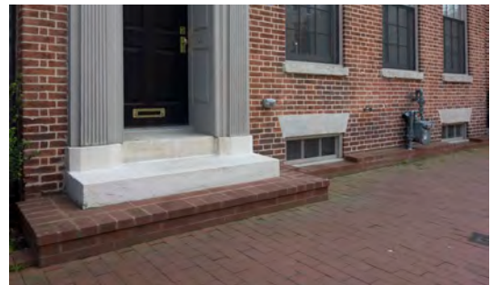
The basement has been abandoned and 1st floor used for parking while maintaining historic appearance.
