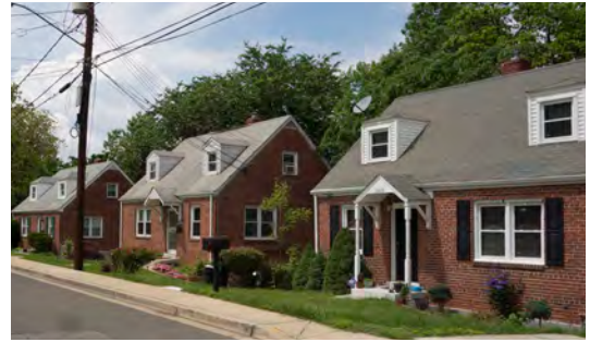
Mid-20th century brick homes are located along Windom and Wallace Roads.
