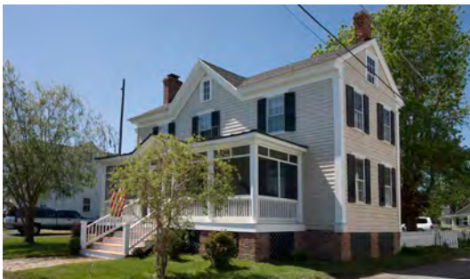
This house was elevated and now includes substantial brick piers. The setback allows a straight-run stair.
