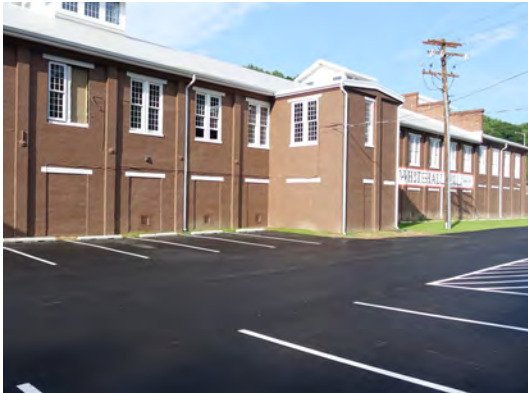
The majority of the ground floor windows were not re-opened as part of the Whitehall Mill rehabilitation, particularly those at the garage.
