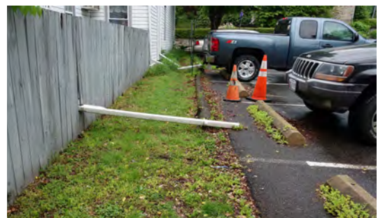
Stormwater drainage from buildings generally discharges to grade.
