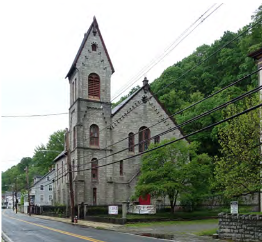
The institutional buildings, including the churches, were typically constructed of masonry, most often local granite.
