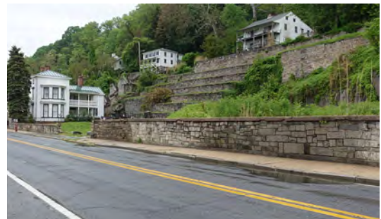
The terraced landscape directs storm water runoff down the hill towards Main Street.
