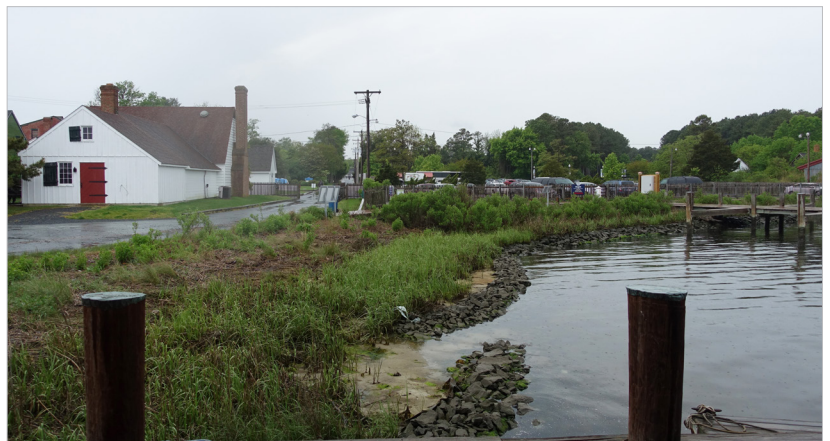
Figure 3.5 - Natural shoreline protection of marsh infill behind small rocks to protect historic buildings. St. Michaels, Talbot County.
