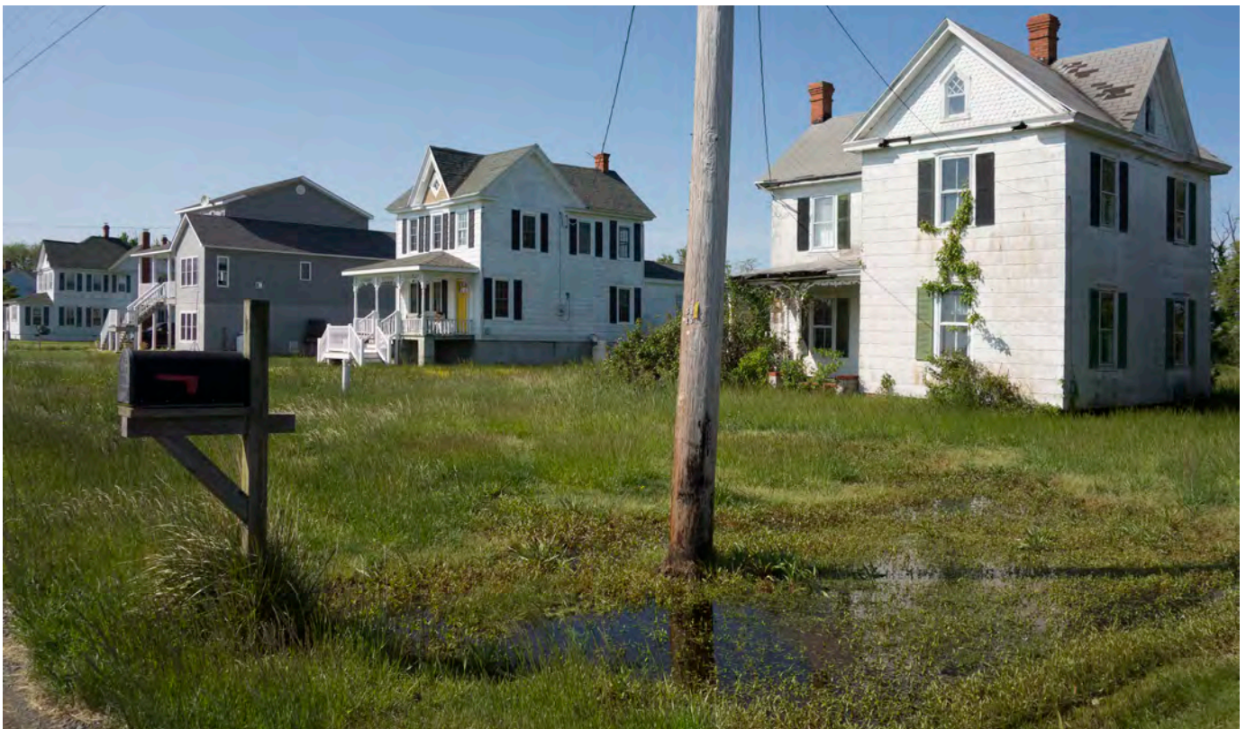
Standing water was present around many of the homes on Hoopers Island, which can cause significant damage to the wood-framed construction, particularly at buildings constructed close to the ground.
