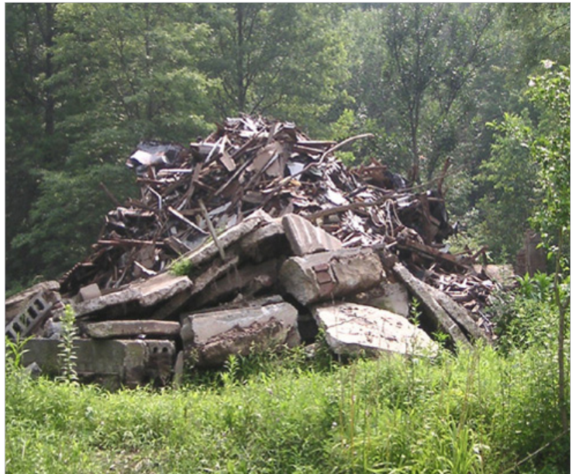
Figure 3.24 - Demolition rubble from a historic cottage.
