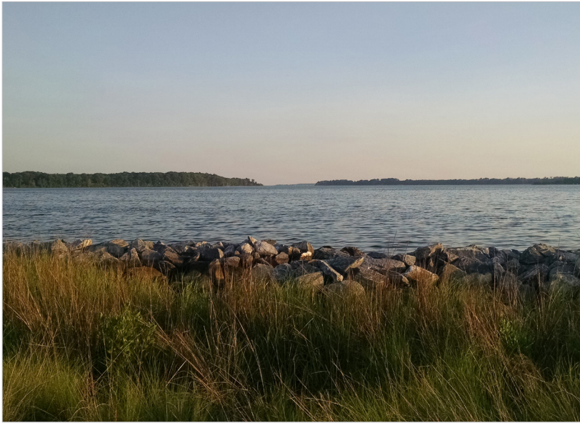
Figure 2.31 - The water's edge includes large rocks (structural shoreline protection) and a marsh (natural shoreline protection), to mitigate erosion along the St. Mary's River and protect the bluffs of Historic St. Mary's City. St. Mary's City, St. Mary's County.
