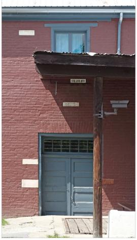
Figure 2.14 - Chesapeake & Ohio Canal Cushwa Warehouse (constructed circa 1790 – 1810) located at the canal's edge has historical high watermarks visible in white block on the face of the building noting the depth of flooding from five food events from the mid-19th to early-20th century. Williamsport, Washington County.
