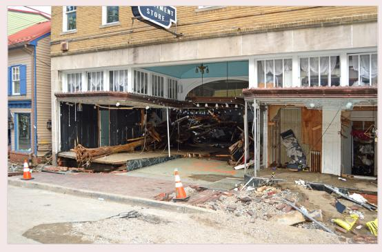
Figure 2.23 - A tree was found lodged in the storefront during initial damage assessments after the 2016 flash flood in Ellicott City. Although the storefront glazing system was lost, its cornice and the transom windows above can be stabilized and retained in the rebuilding process.
