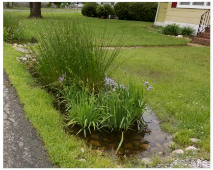
*Figure 2.32 - Rain gardens provide an efficient means of minimizing stormwater runoff and can often be integrated into existing landscaping. Shady Side, Anne Arundel County.*
