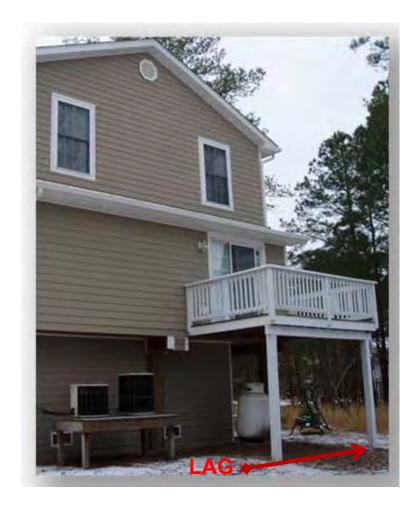
Figure 2: LAG - Structure with Attached Deck
