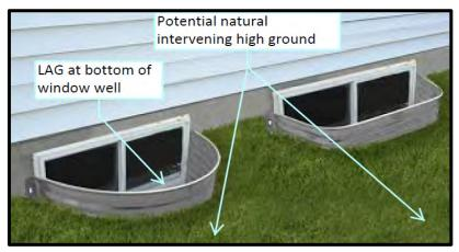
Figure 20: Use of Intervening High Ground – Window Well
