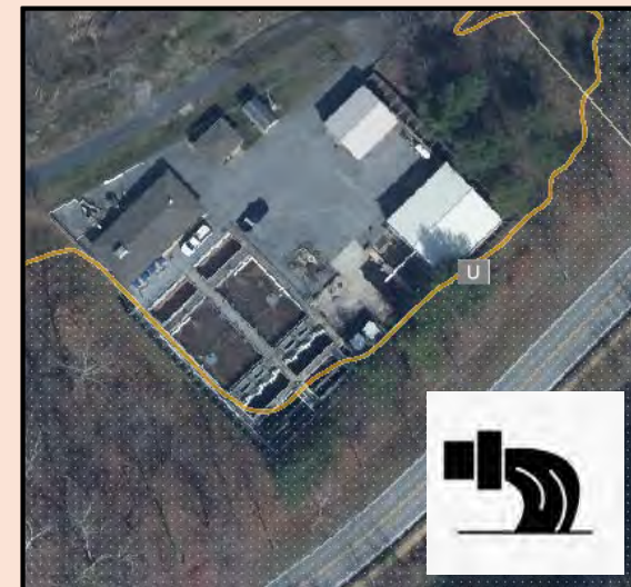
Harpers Ferry Bolivar PSD Wastewater Treatment Plant (FD: 1 ft) (Building ID: 19-05-0004-0025-0000_192 ) ($462K) Value source inflation adjusted to 2021
