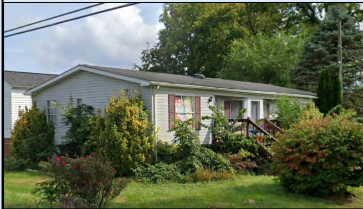
Double-wide Mobile Home in Ranson (FD: 2.2 ft) $33K; Year Built: 1993 (Post-FIRM) (Building ID: 19-08-0006-0019-0001_407 )
